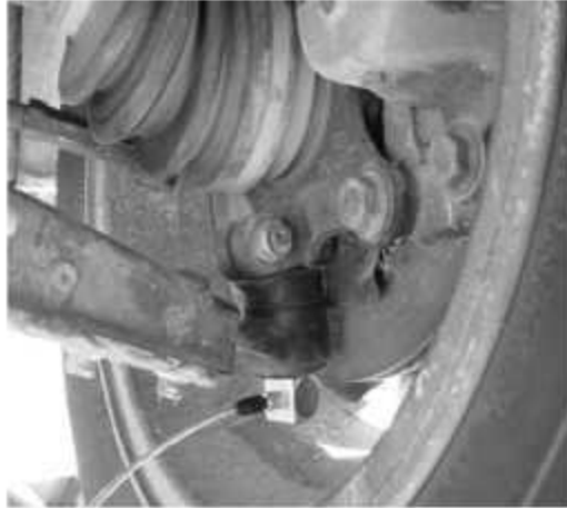
Figure 52. Bolt damage location.
