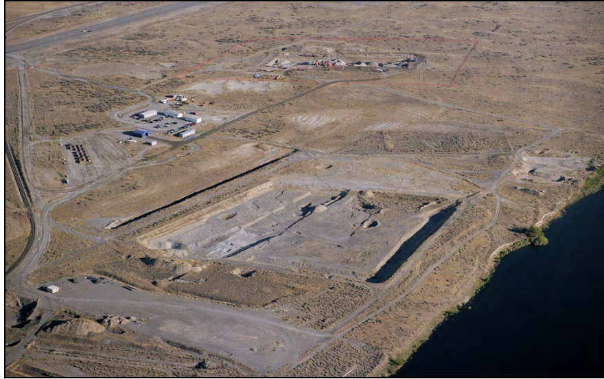
Figure 6.6. Aerial Photo of North Process Pond Open Excavation. Date of photo is prior to excavation of 618-5 burial ground, which started in October 2002.
