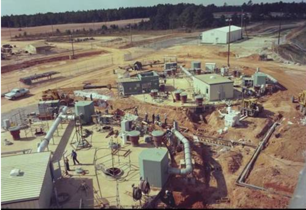
Fig. 1. SRS Tank Transfer Piping Construction
