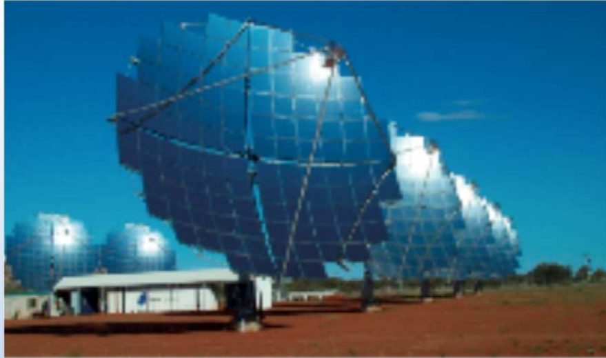
Large dish: Stirling engine; PV requires active cooling
