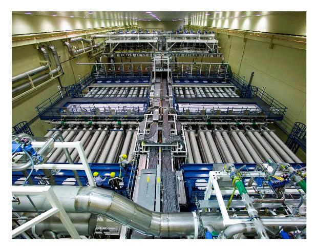
**NIF Laser Bay** – This is one of NIF's two laser bays. This room is the about the length of a football field and contains grouped beampaths that transport 96 laser beams through a four-pass amplifier system and spatial filtering chambers and then send the beams to the target chamber. Vacuum, gas, water and other utility systems have been installed to provide tightly controlled environmental conditions to assure that each laser beam meets the specifications required for NIF experiments.
