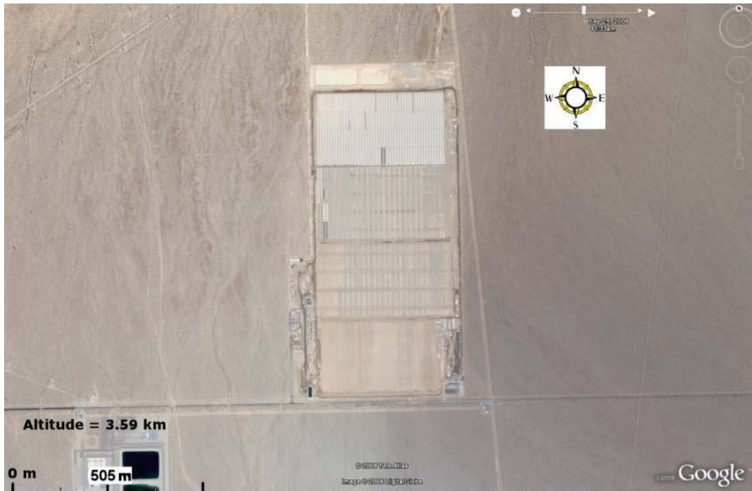
Figure B-4. Image of NSO solar power plant in Boulder City, NV, obtained from Google Earth
