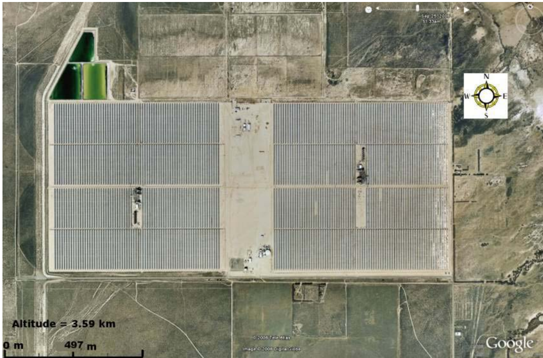
Figure B-3. Image of SEGS VIII (left) and IX (right) solar power plants in Kramer Junction, CA, obtained from Google Earth
