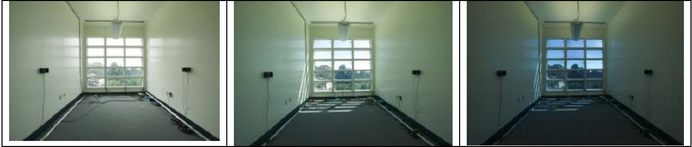
Figure 3 New LBNL facility for comparative field tests of advanced facades. Electrochromic glazings are controlled real-time to meet design illuminance but control solar gain and glare. Left: Under cloudy conditions the glass is at maximum transmittance. Center: When sun comes out the window begins to darken. Right: After 5 minutes the window is fully darkened but the lights are on to meet illuminance levels.
