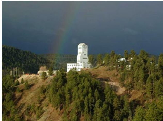
Figure 1: Homestake Mine Headhouse
