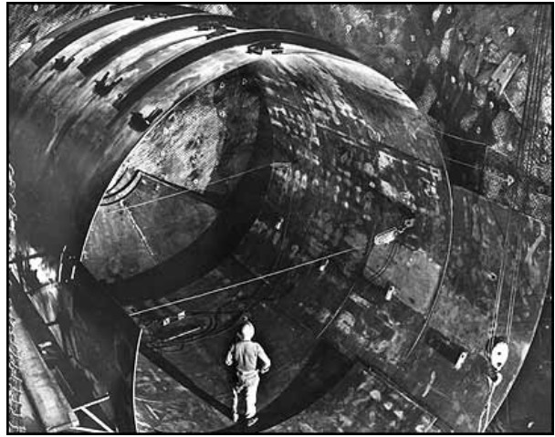
Figure 3: Homestake's First Neutrino Detector (Source; Brookhaven National Laboratory)
