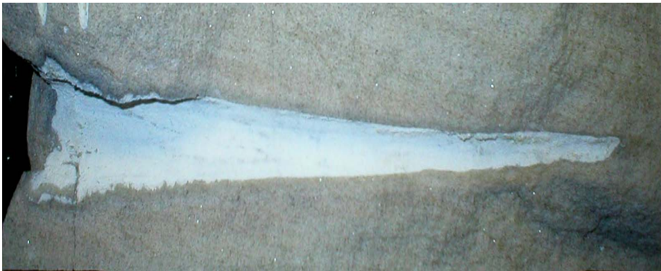
Figure 119. Deep hole in limestone of 12 inches deep.
