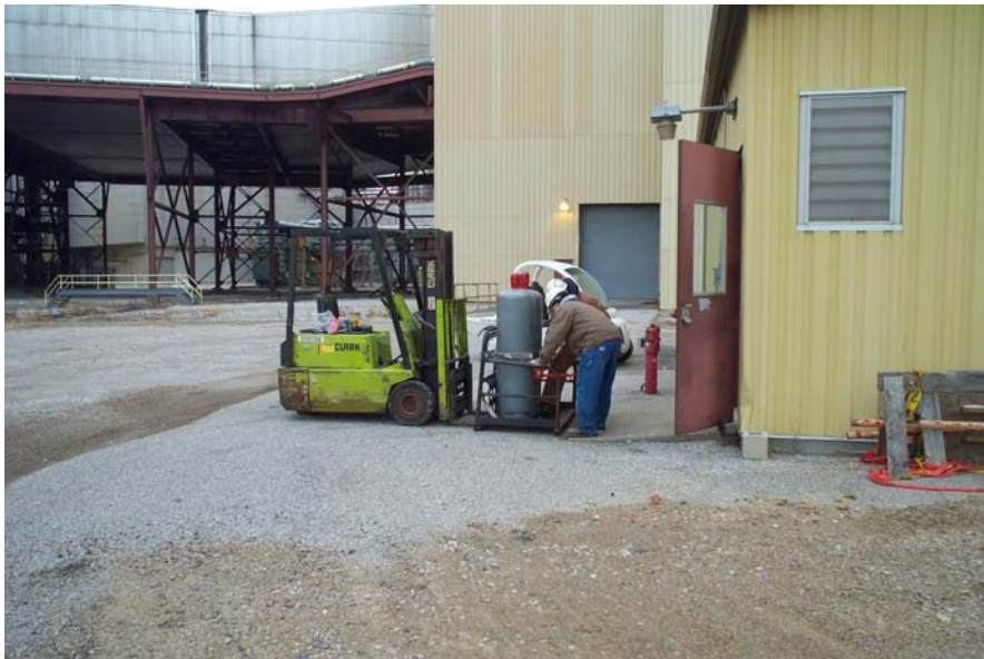
Figure 5.76. Ammonia cylinders being prepared for hauling to the installation site.
