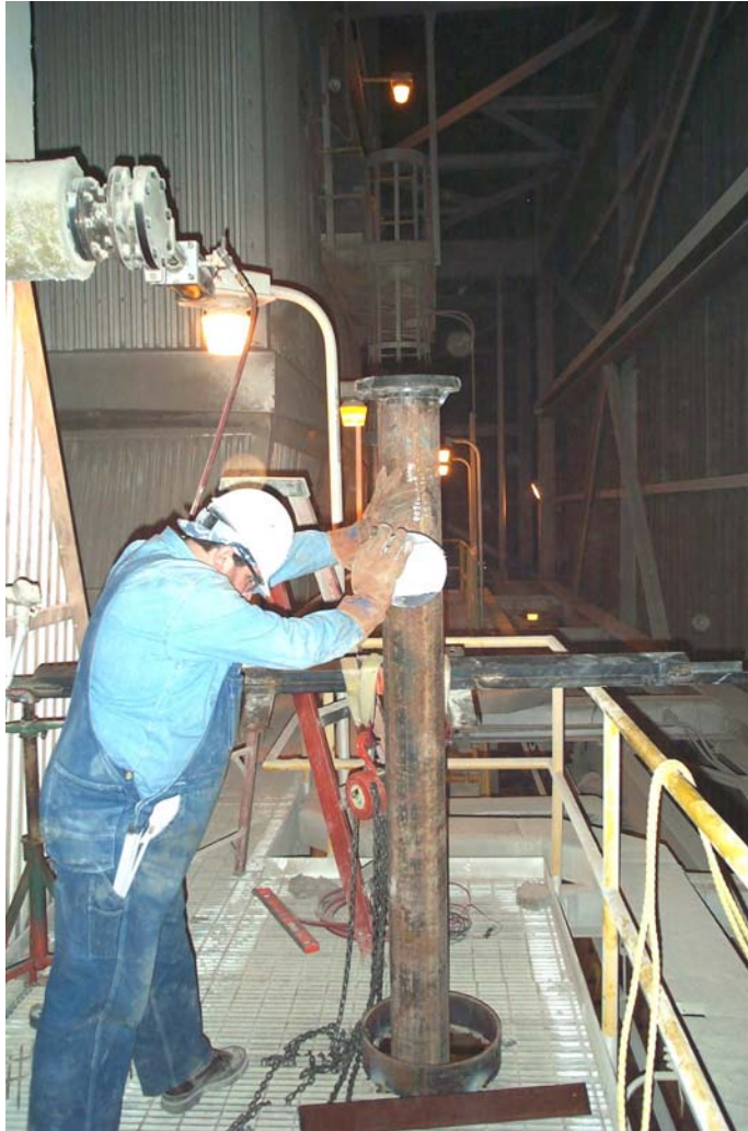
Figure 5.73. Installation of the SCR flue gas intake pipe at Rockport.
