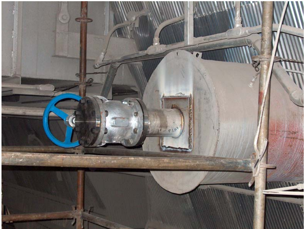
Figure 5.92. Outlet port installed at air preheater exit at Plant Gadsden.
