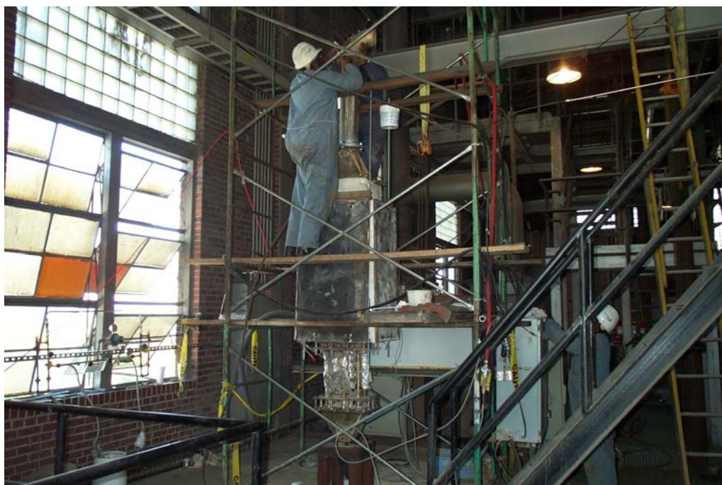
Figure 5.93. Assembly of slipstream reactor.
