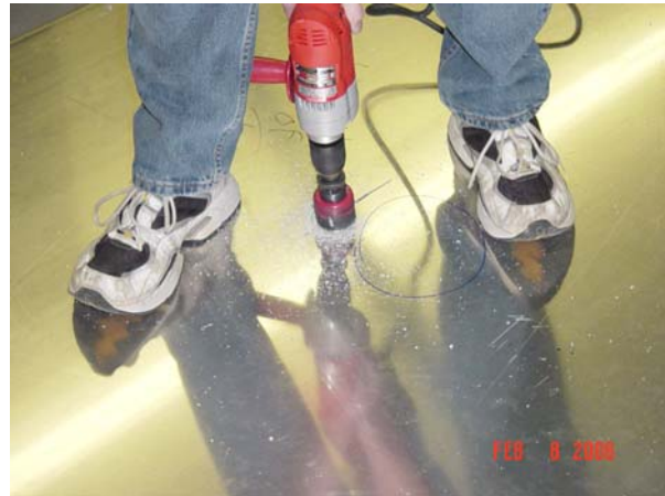
Figure 6.4. Bypass hole drilling.
