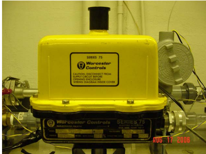
Figure 6.12. Motor-operated valve (MOV) electric actuator.
