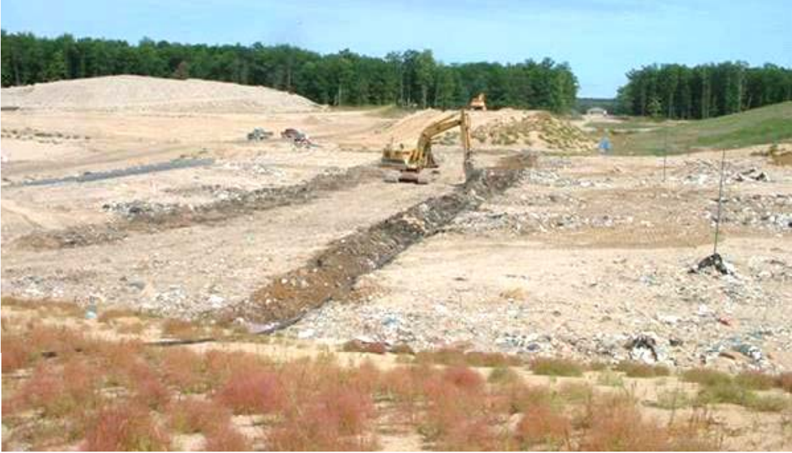
Figure 6-6: Installation of settlement profiler conduits
