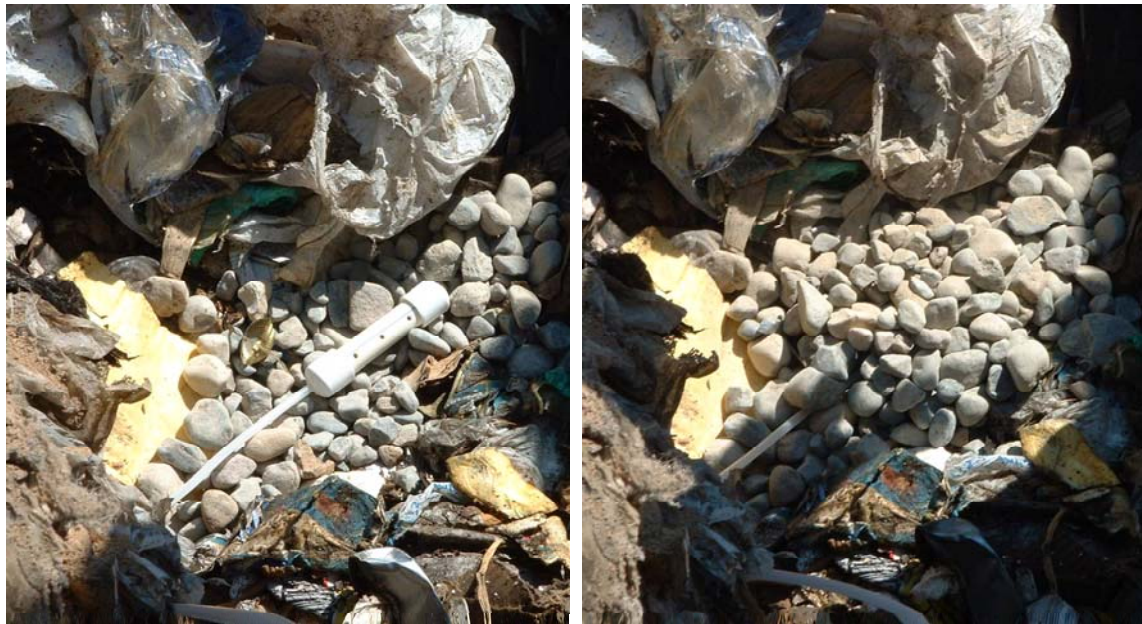
Figure 6-5: Installation of the gas sampling port
