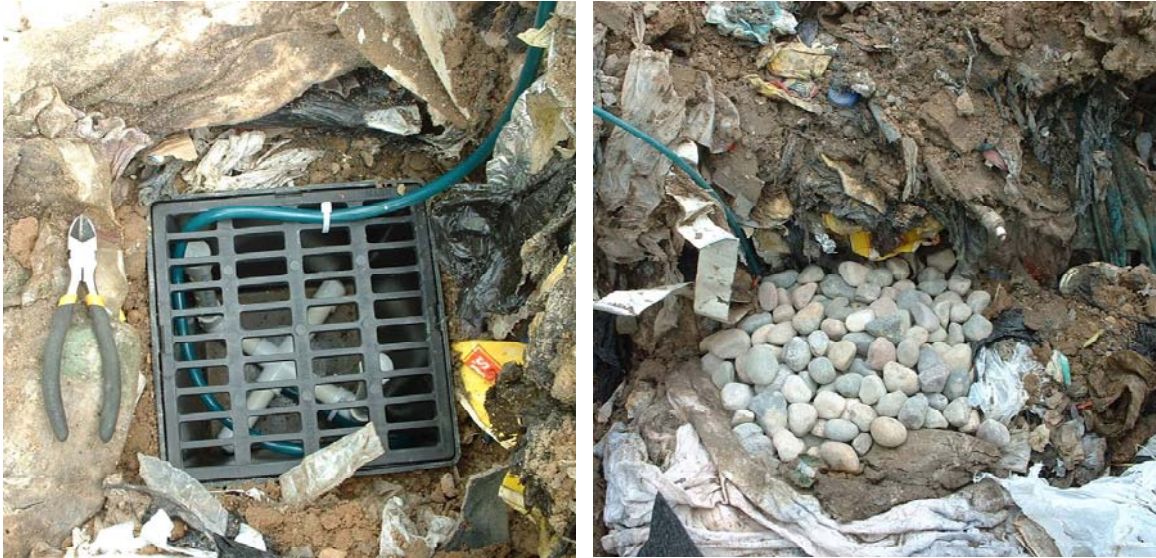
Figure 6-4: Installation of the leachate collection basin
