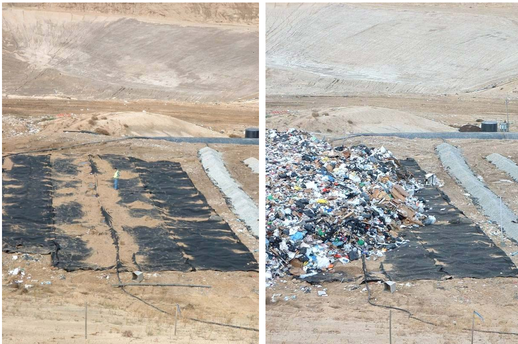
Figure 4-7: 60-ft wide geocomposite leachate distribution layer
