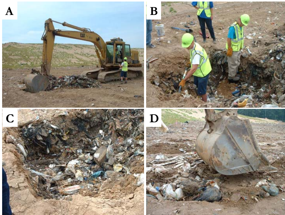
Figure 6-2: Placement of in-situ monitoring instruments at selected locations
