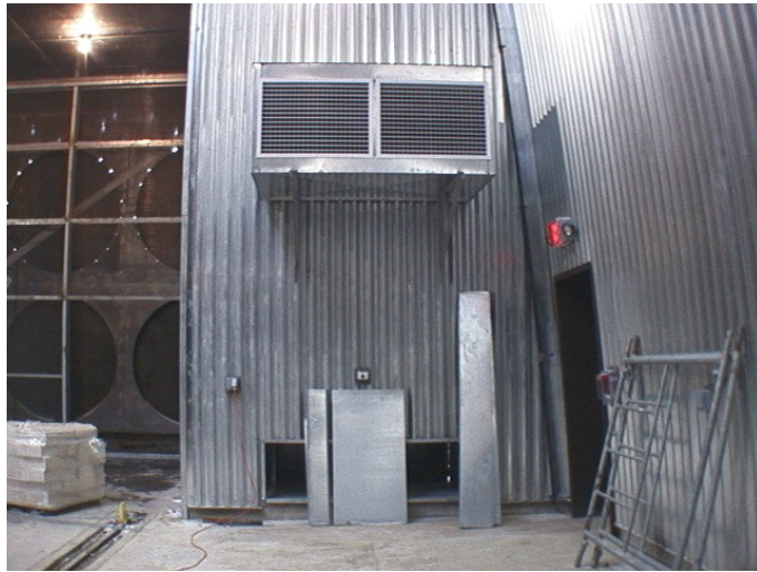
Figure 2-9 The heater mounted on the upstream wall during construction
