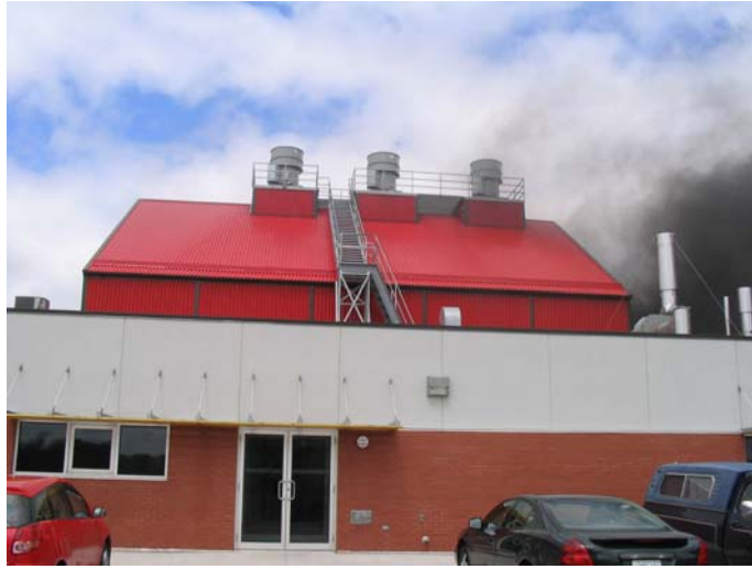
Figure 2-6 A view from the south of the LFRF during a fire test
