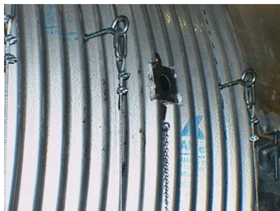
b. Eyehooks mounted to the C/MF
