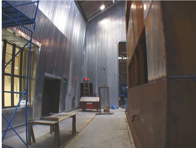
Figure 2-10 A view of the south side of the LFRF looking upwind with the house test cell installed
