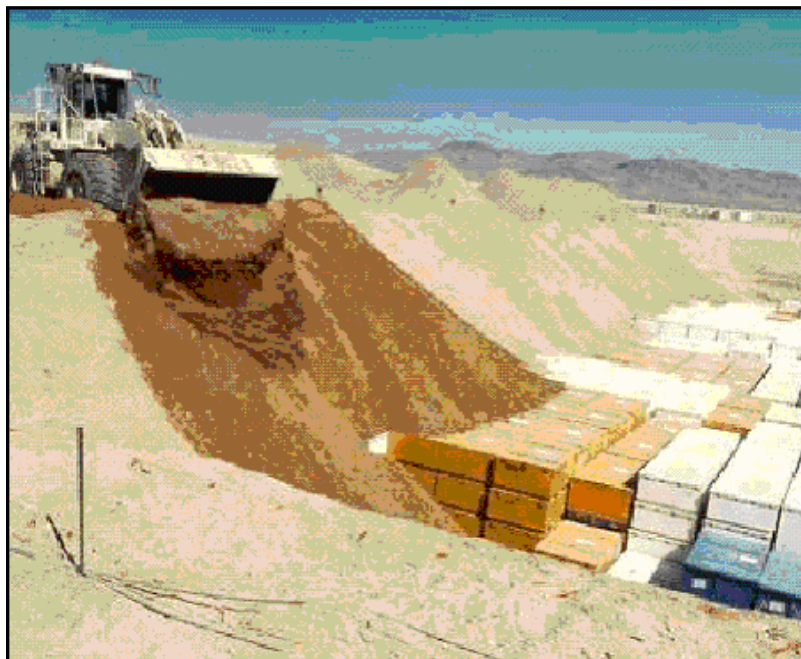
Figure 3-2. Placement of Backfill Over Waste Containers
