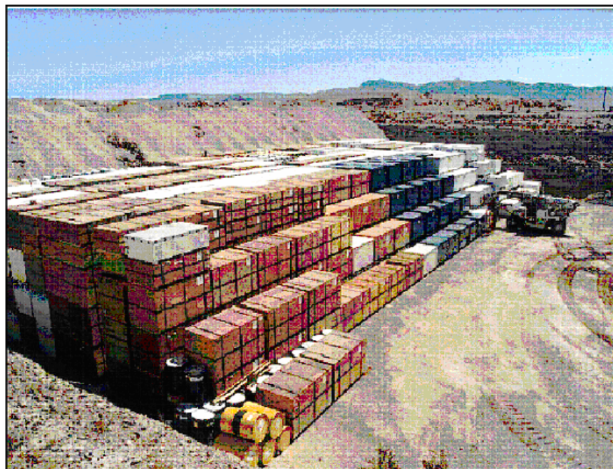
Figure 3-1. Waste Container Placement in a Typical Pit at the Area 5 Radioactive Waste Management Site
