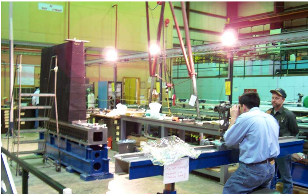
Figure 6, the optical transit in use aligning a submodule on the support girder.
