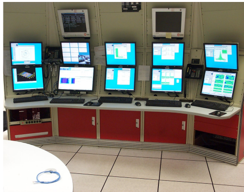
Section of the CDF control room at Fnal devoted to the Consumer Monitors
