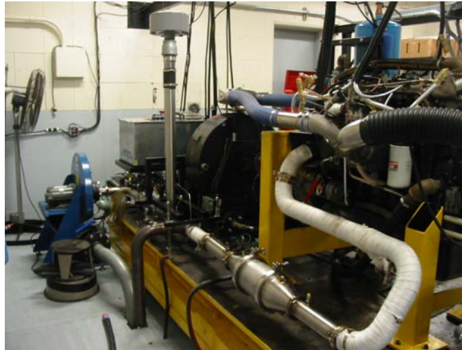
Figure 5.6. Prototype trap installed in the ISB exhaust system
