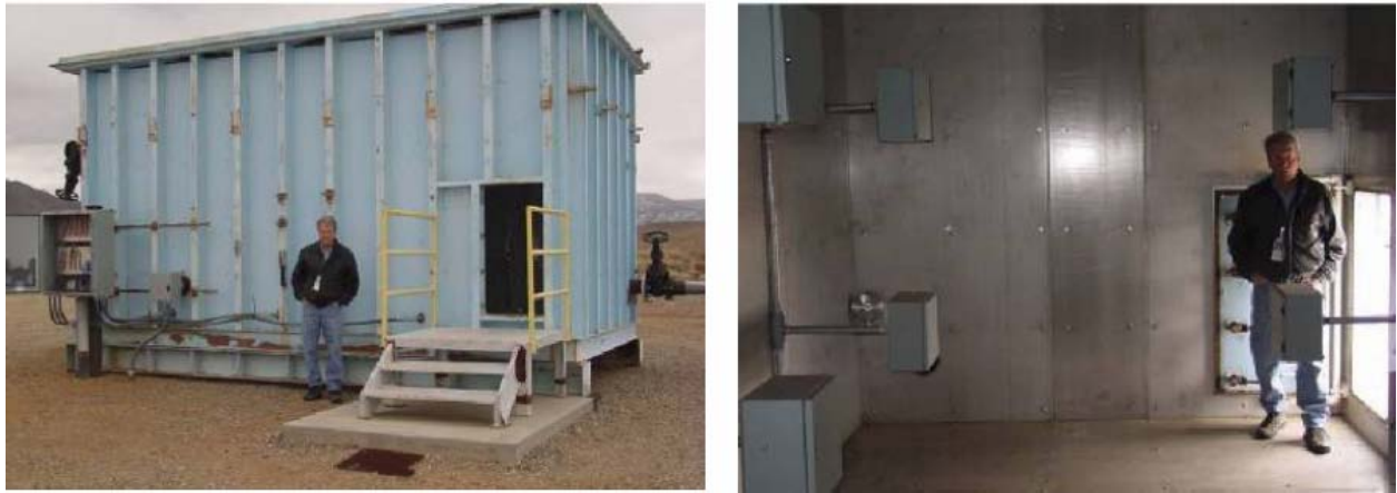
Figure 3.1.1. SNL Site 9920 50 m 3 Steel Test Chamber, External and Internal
