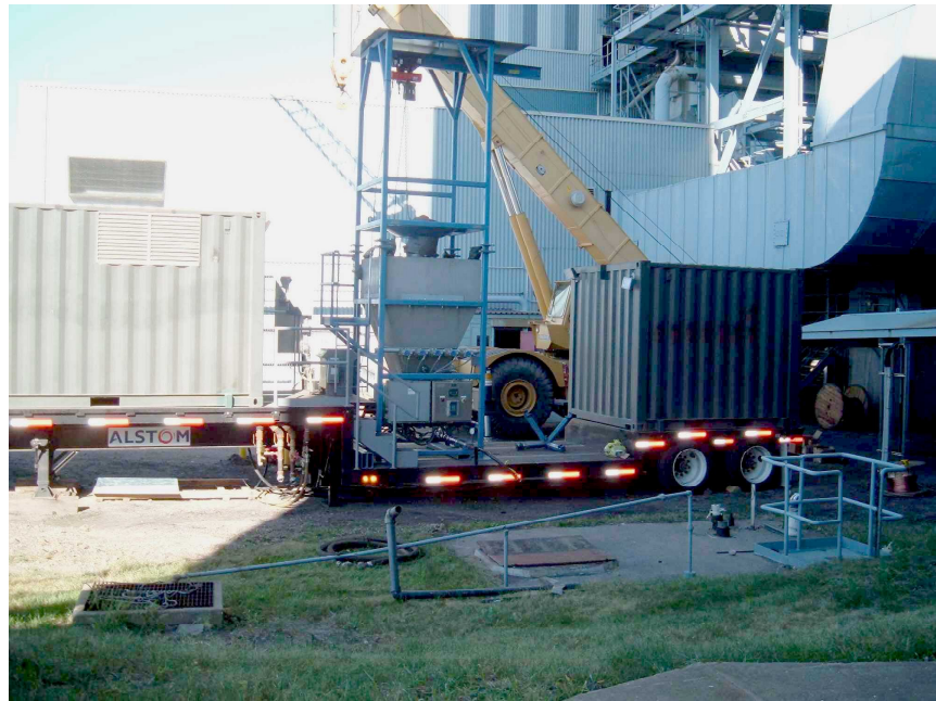
Figure 4.2-3 On Site Assembly of Mobile Mer-Cure™ Demonstration Trailer
