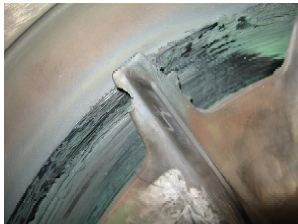
Figure 47: Close-up of Turbine blade damage
