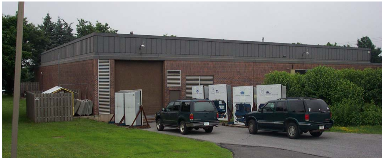
Rear of Building (West)
