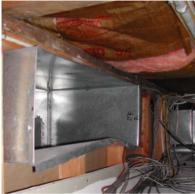
Typical supply diffuser
