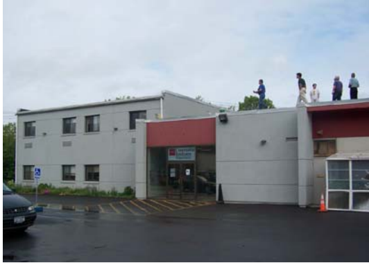
Main Entrance (Site 15, south)
