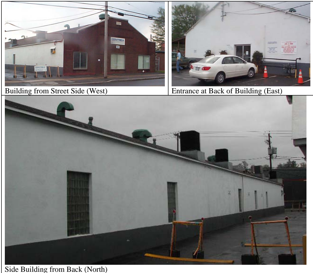
Figure A4-1. Photos of Building
