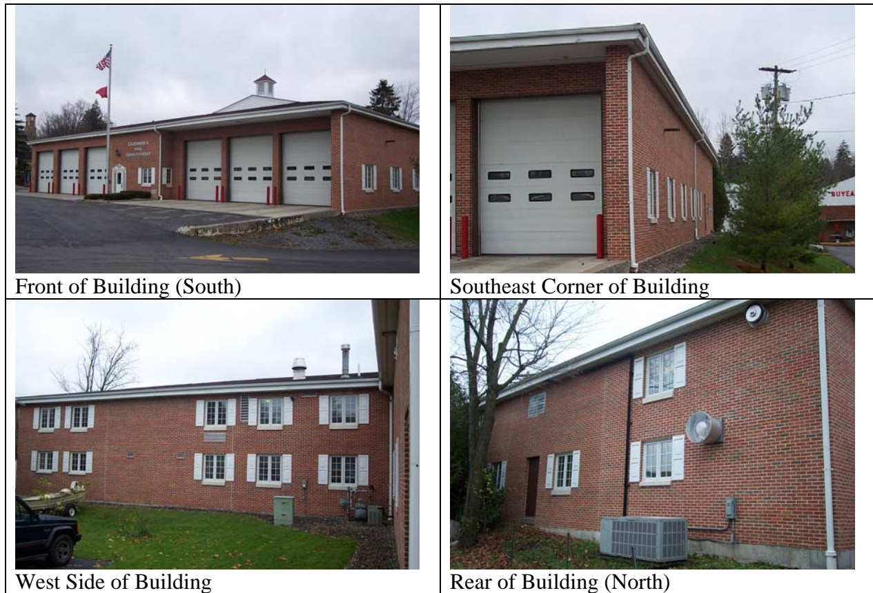
Figure A13-1. Photos of Building
