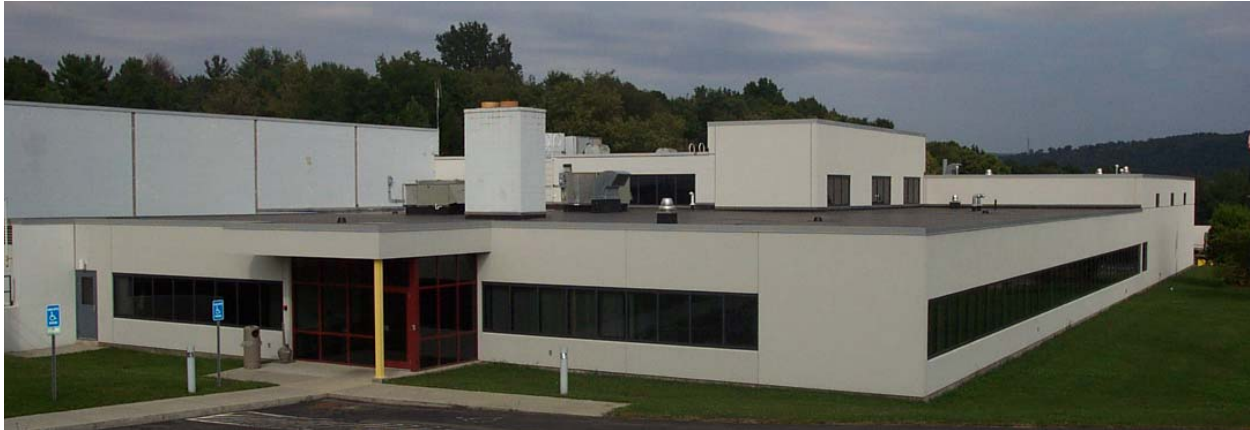
Figure A10-1. Photo of Building (Southwest)
