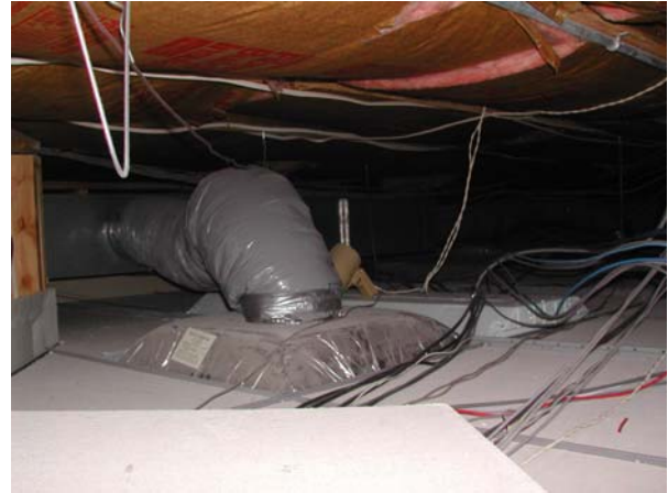
Typical supply diffuser
