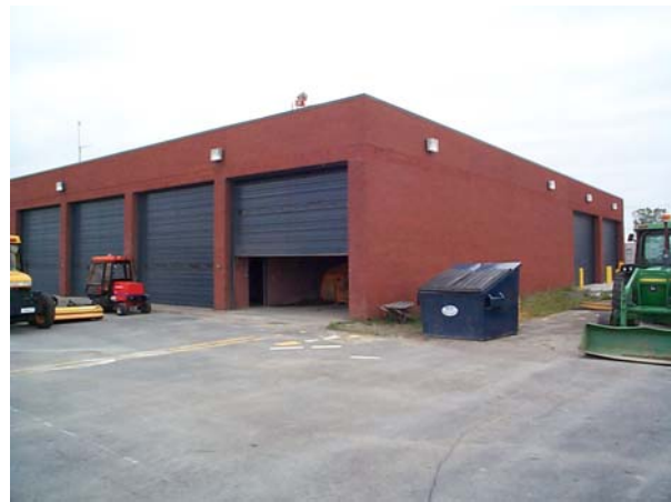
Back Side of Building (North Corner)
