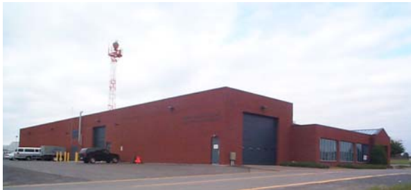
South Corner of Building
