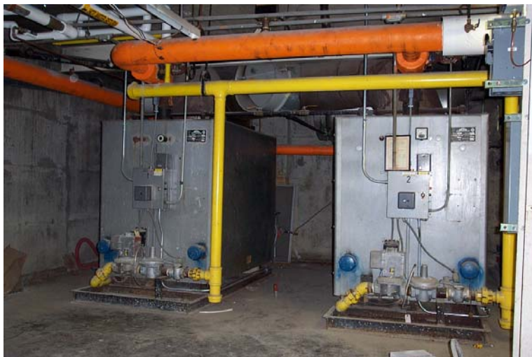
Figure A10-9. Hot Water Tube Boilers
