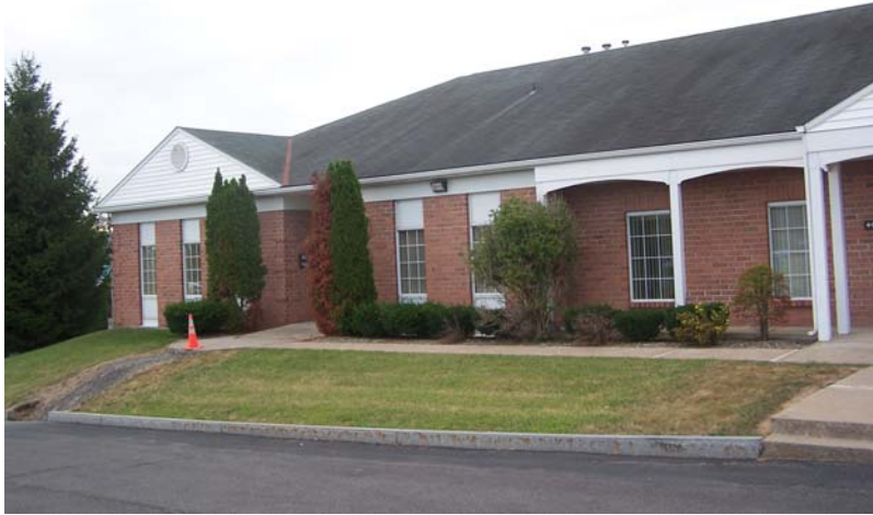
Main Entrance (North)
