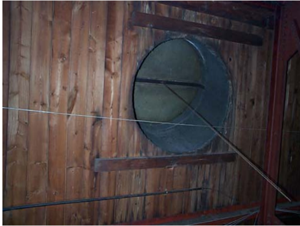
Attic Vent through Roof Decking (Closed)
