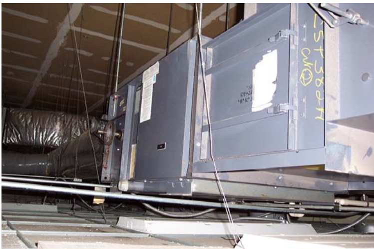
AC-2 (Cooling Only) Trane Climate Master, Unit Type: CCDB03AB0J, Basic Unit: H3A1R01L0AF
