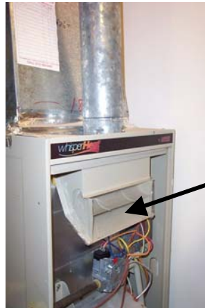
Furnace Exhaust Vent (1 of 8)
