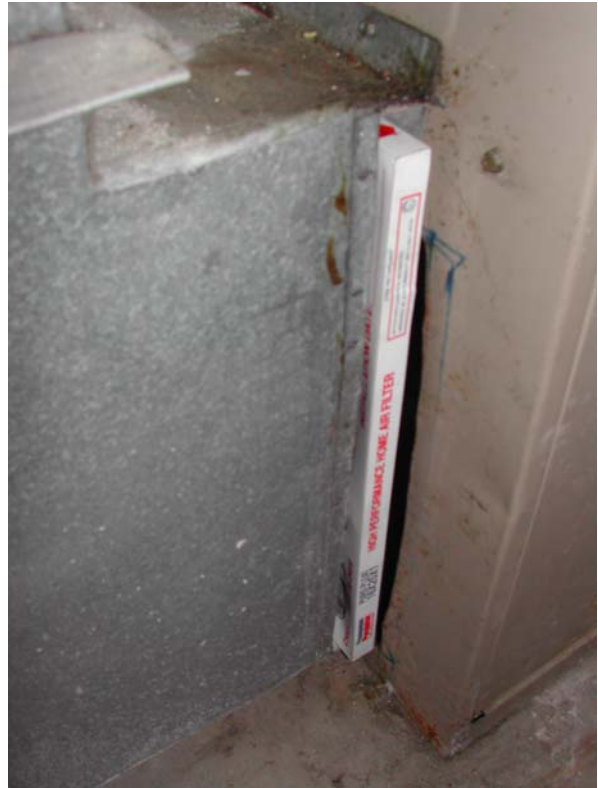
Furnace, Ductwork & A-coil - East
