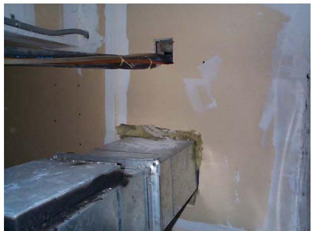
Ceiling Plenum Interior Wall
