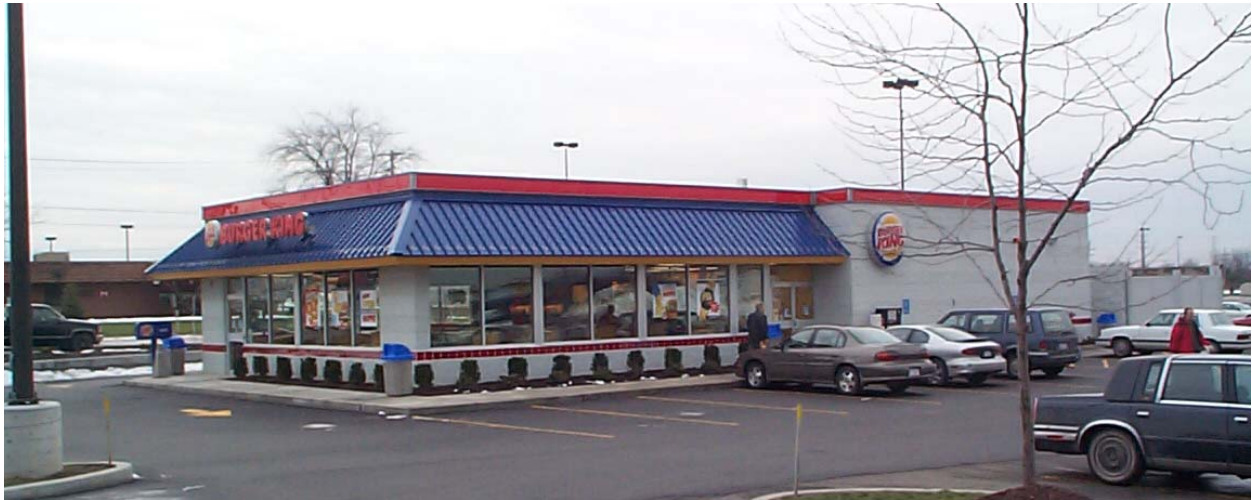
Figure A9-1. Photo of Building (Northeast)
