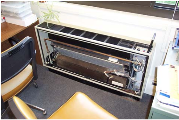
Console PTAC with Front Cover Off
