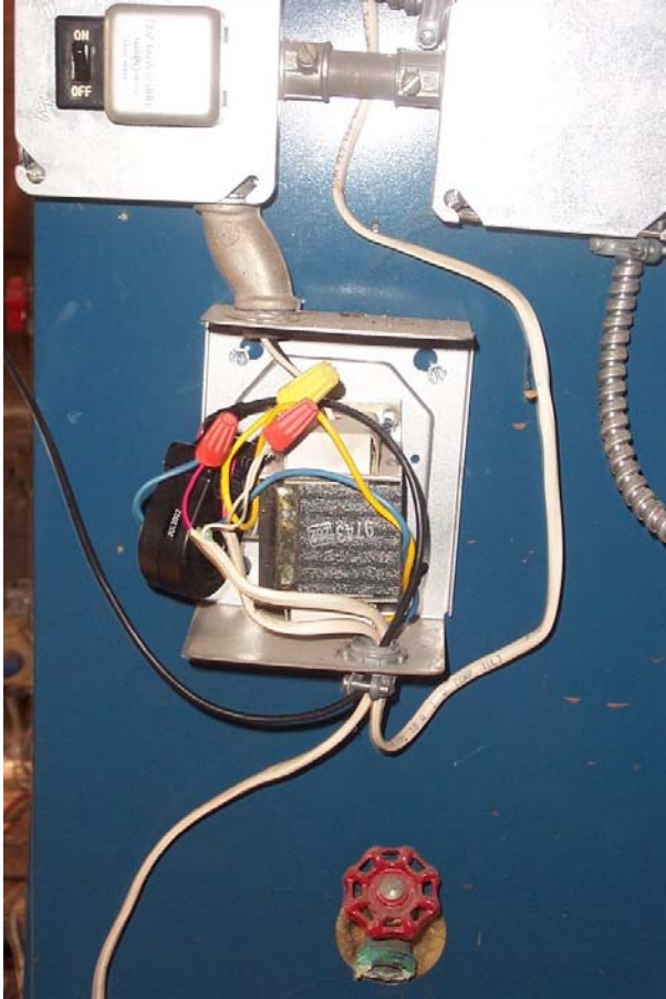
Figure A17-34. Current Status Switch on 24 VAC Control Transformer for Boiler Natural Gas Train
