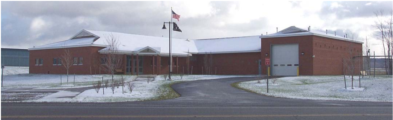
Main Entrance (Southwest)
