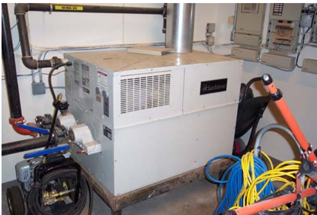
Figure A12-7. Hot Water Boiler and Cooling Towers to Maintain Water Loop Temperature
