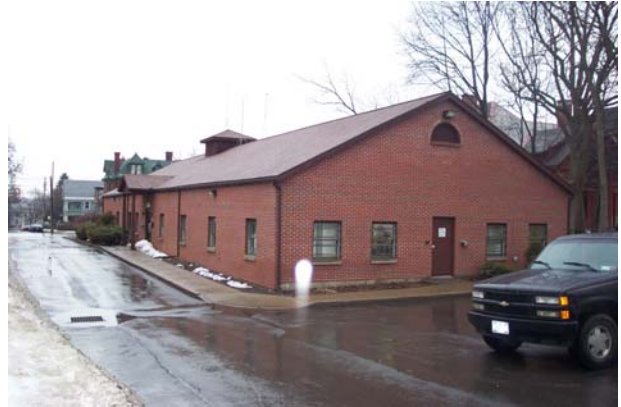
Building from the Rear (east)
