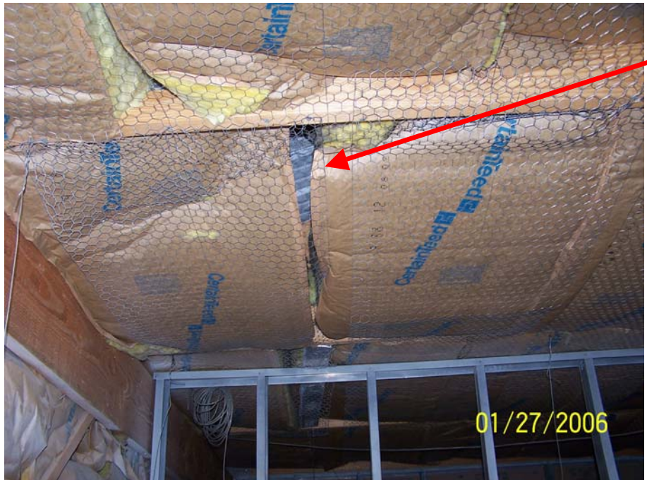
Insulation held up by Chicken Wire (gaps exist in insulation)
