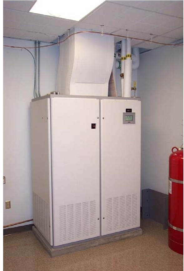
Constant Volume Unit (AHU-3) Canatal Model: 8CU10
