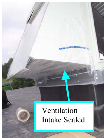
Ventilation Hood Sealed
