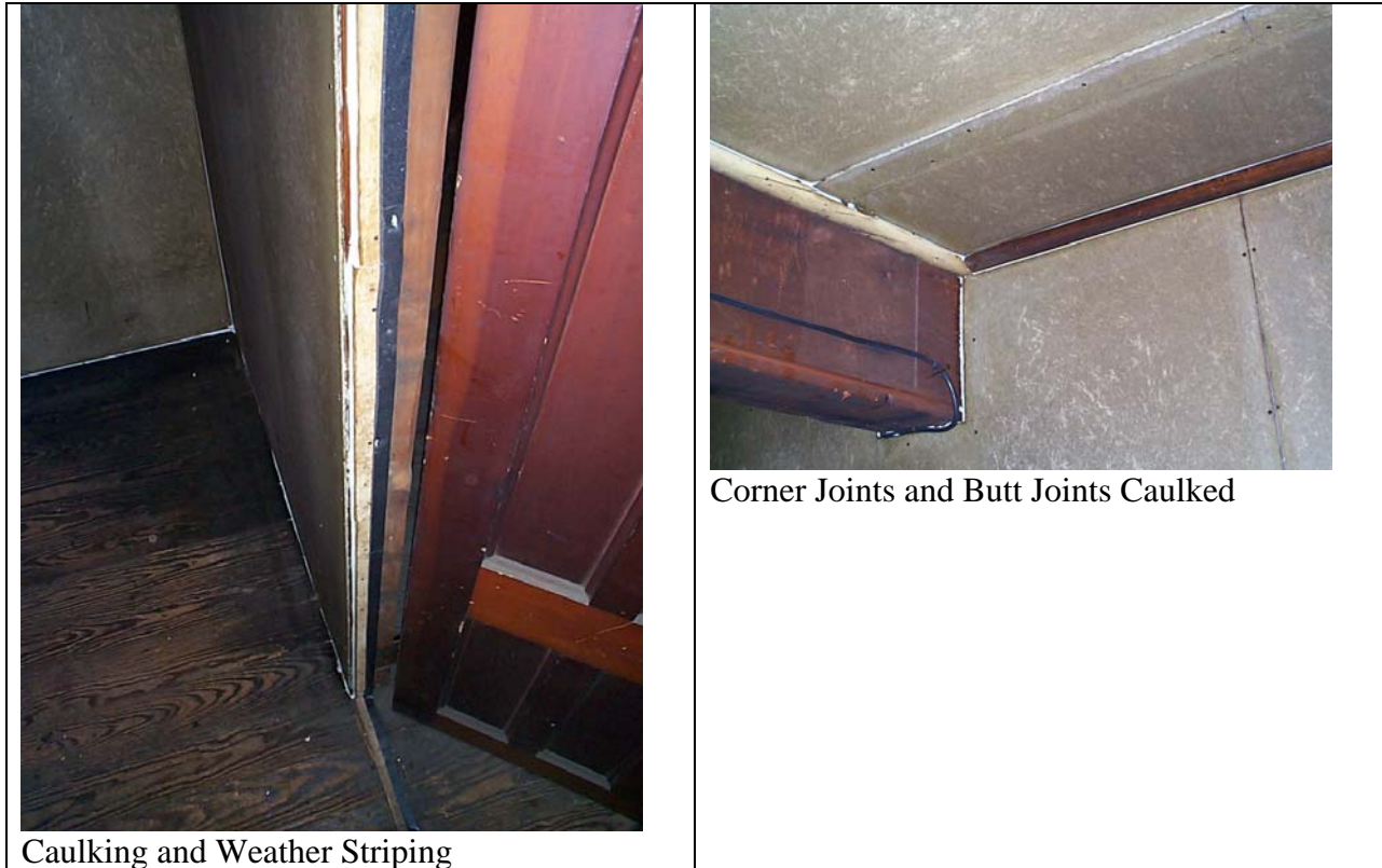
Figure A17-33. Sealing the Elevator Mechanical Room
