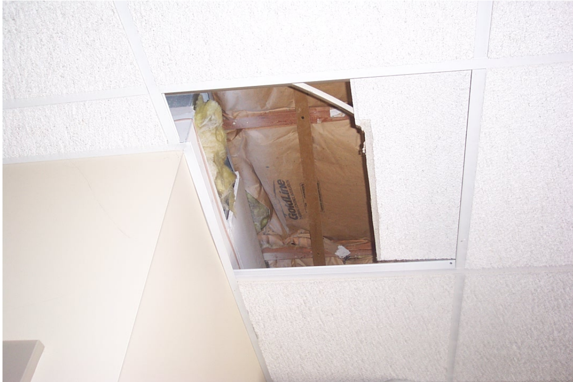
Figure A2-33. Furring Strip Installed to Support Batts
