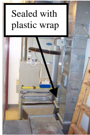
Fresh Air Vent for Upstairs Furnaces (1 of 2)
