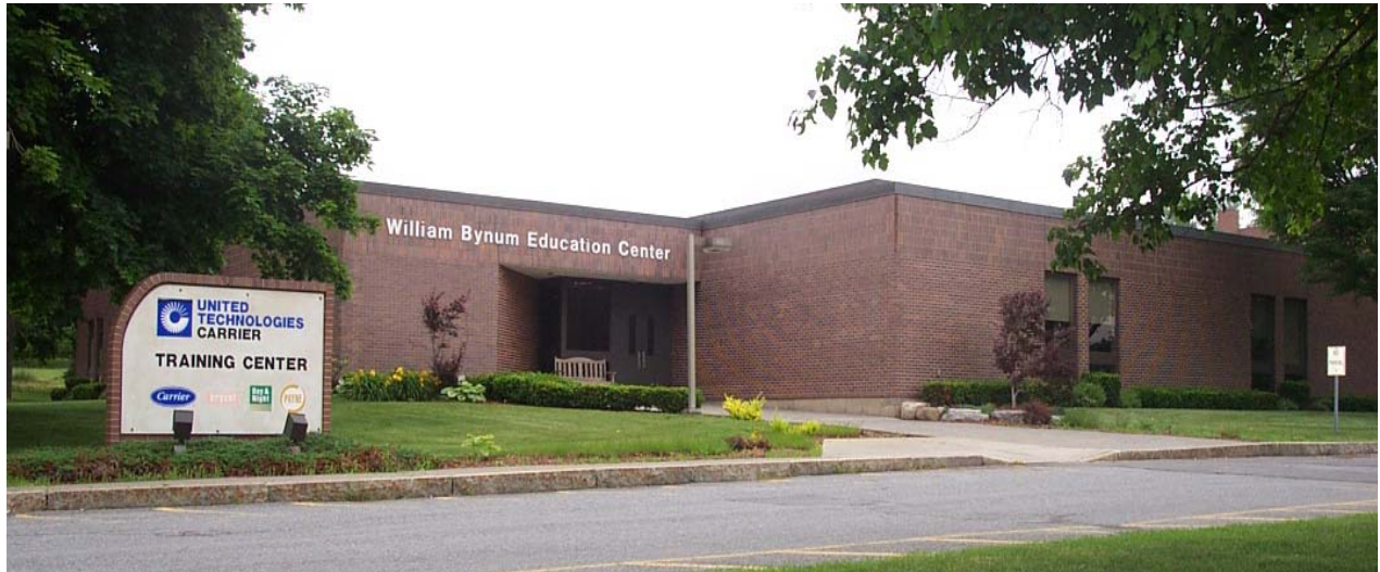
Front of Building and Main Entrance (East)
