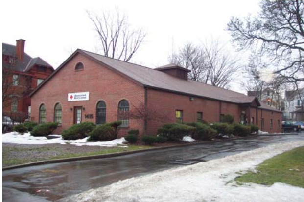
Building from the Front (west)
