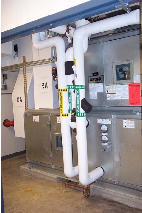
VAV Unit (AHU-1 & AHU-2 are identical) York Model: AP-105 Coil Model: BA0060830.00x048G01HB016S032WH02R Coil Model: CA0061230.25x048G08CC020S035WH16R
