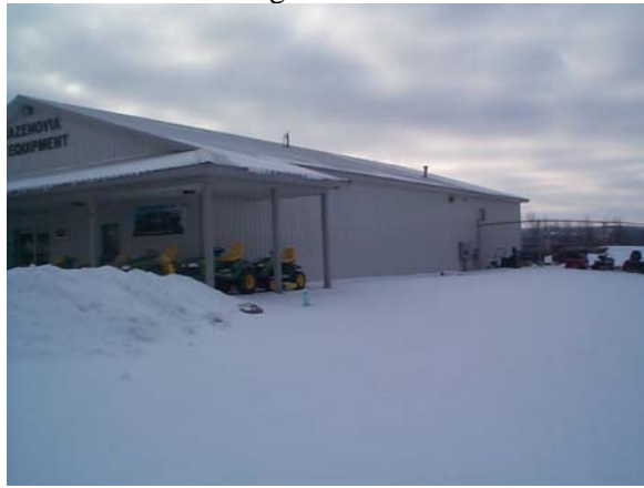
West Side of Building
