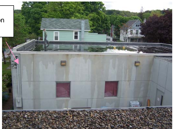
Front of Ag Building where EFIS stops near meter
