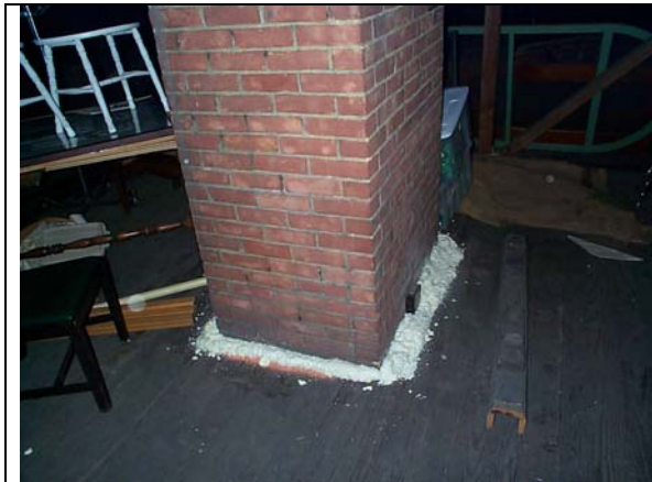
Around Chimney Penetration
