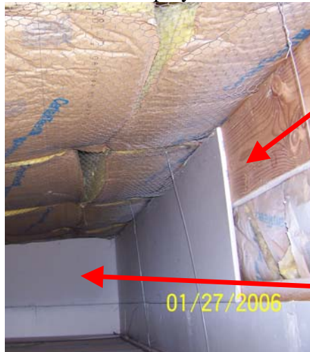
Insulation held up by Chicken Wire (gaps exist in insulation)
