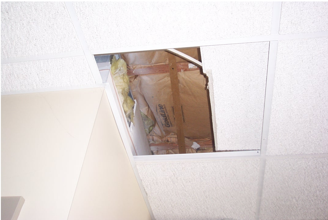
Figure 3-5. Furring Strip Installed to Support Fiberglass Batts from Underneath
