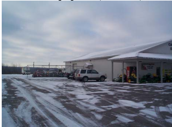
East Side of Building
