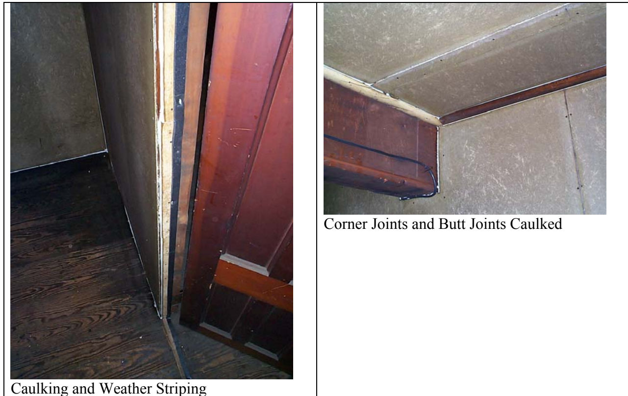
Figure 3-18. Sealing the Elevator Mechanical Room in Attic at Site 17
