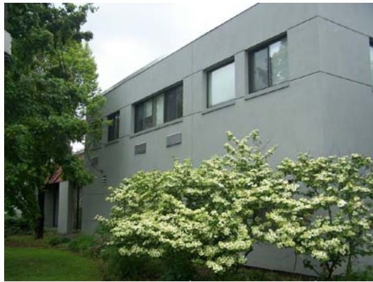
Street Side of Willow Building (Site 15, north)
