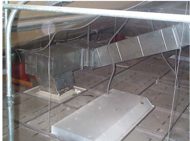
Typical Diffuser Installation
