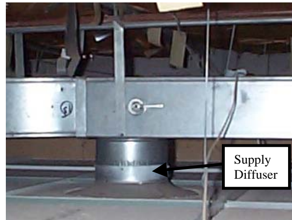
Typical Supply Diffuser Installation
