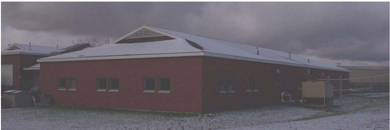
Rear of Building (Northeast)
