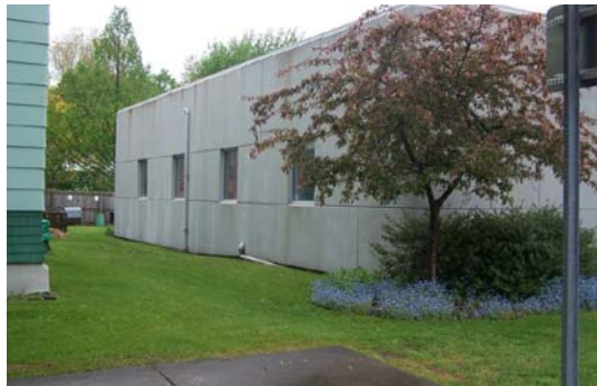
East Side of Ag. Building (Site 16)
