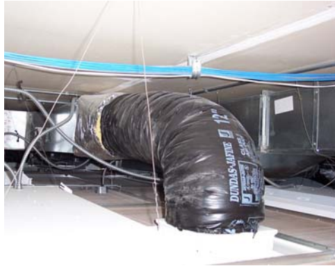
Typical Diffuser Installation
