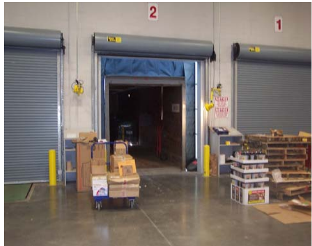
Loading Dock Doors on West Side of Building
