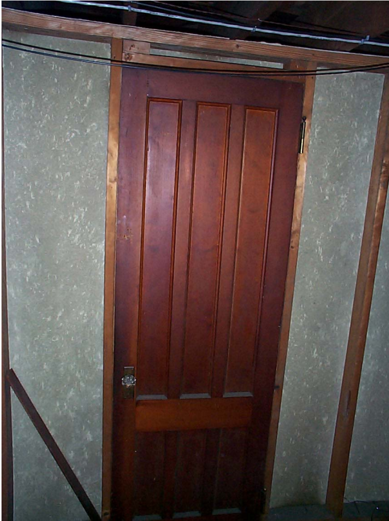
Figure A17-30. Exterior of Elevator Mechanical Room (Viewed from Attic)
