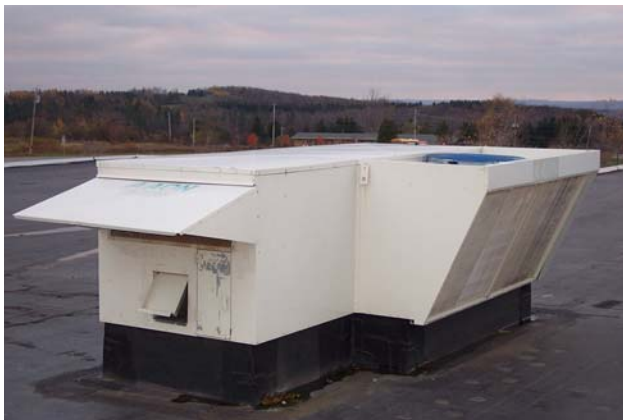
Figure A12-6. Aeon 3-ton Rooftop with Enthalpy Wheel Unit
