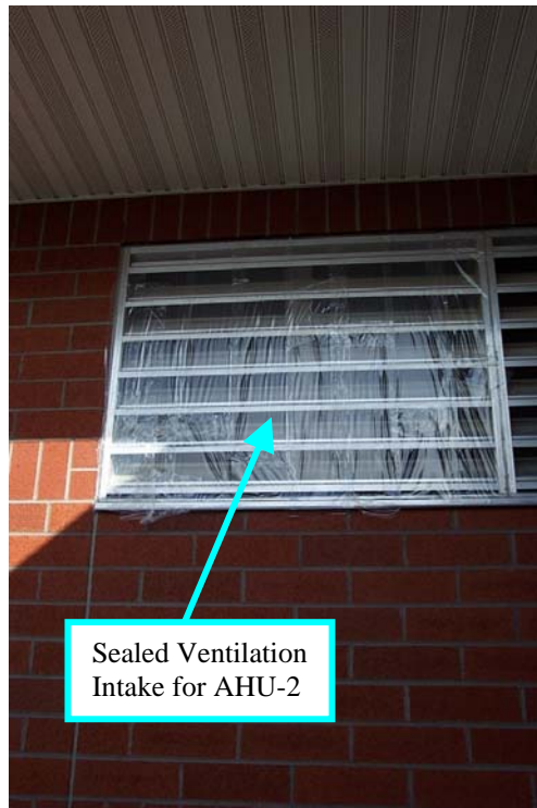
Seal Isolating Supply & Return Ductwork AHU-2 Ventilation Intake
