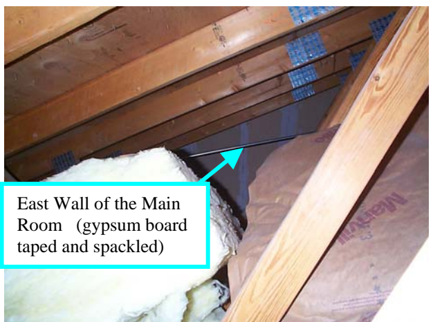
Figure A8-5. Attic Type Space between the Roof and Primary Air Barrier
