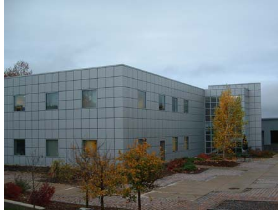
Rear of Building (Northeast)
