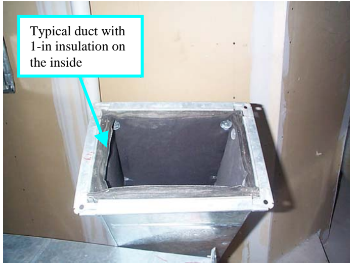
Figure A8-7. Insulated Ductwork
