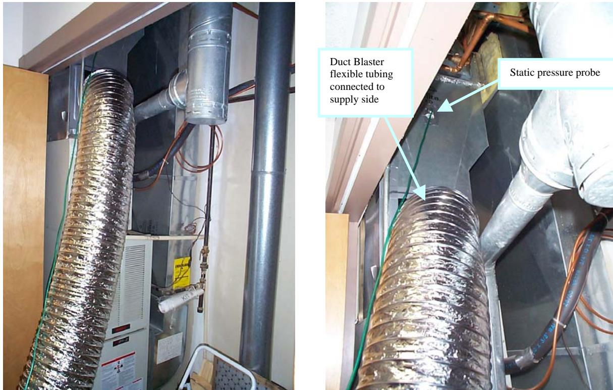
Figure A2-17. Duct Blaster Setup for Duct Leakage Test
