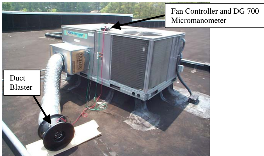
Duct Blaster Set Up to Measure RTU Ventilation
