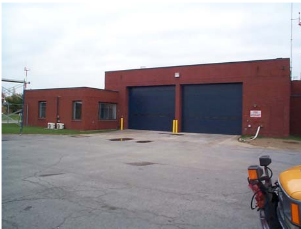
Back Side of Building (East Half)
