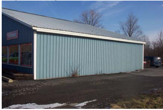
West Side of Building
