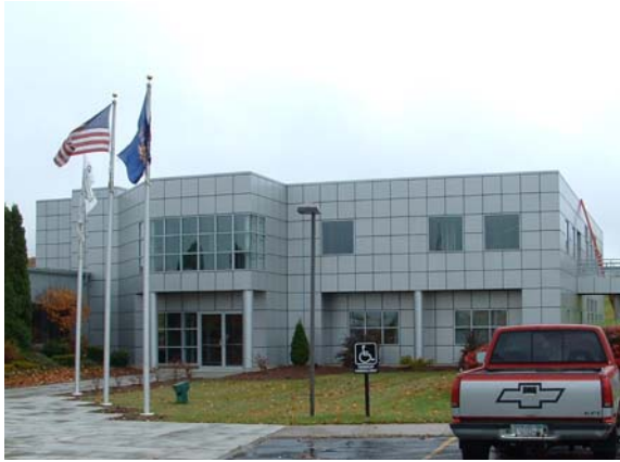
Main Entrance (South)
