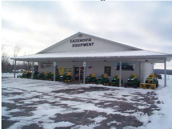
Main Entrance (North)
