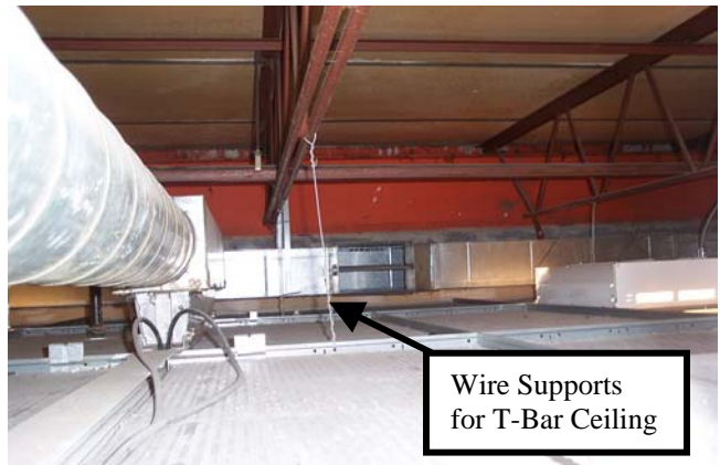
Ceiling Plenum in Classrooms and Offices
