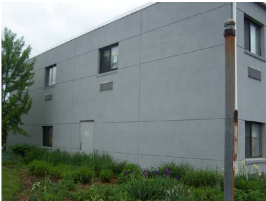
West Side of Willow Building (Site 15)
