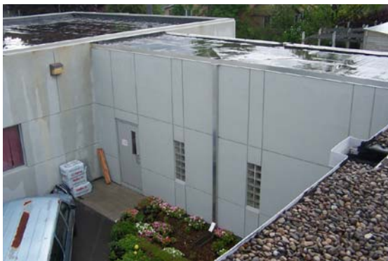
Connection Hallway (north)
