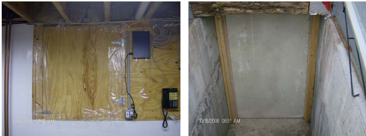
Figure A25-12. Basement Half Door Tapped Off (Left) and Exterior Basement Door (added for Tests 6 & 7)
