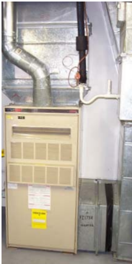
Lennox Furnace (F3) Model: G20Q3/4E
