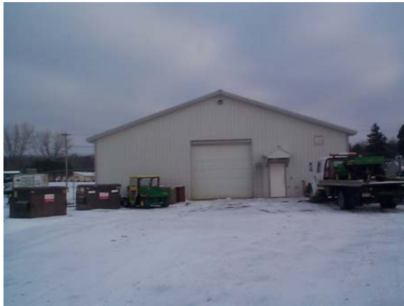
Rear of Building (South)
