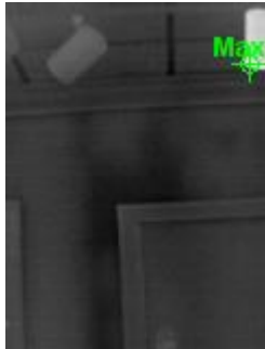
Wall Void Behind Electrical Service Entrance
