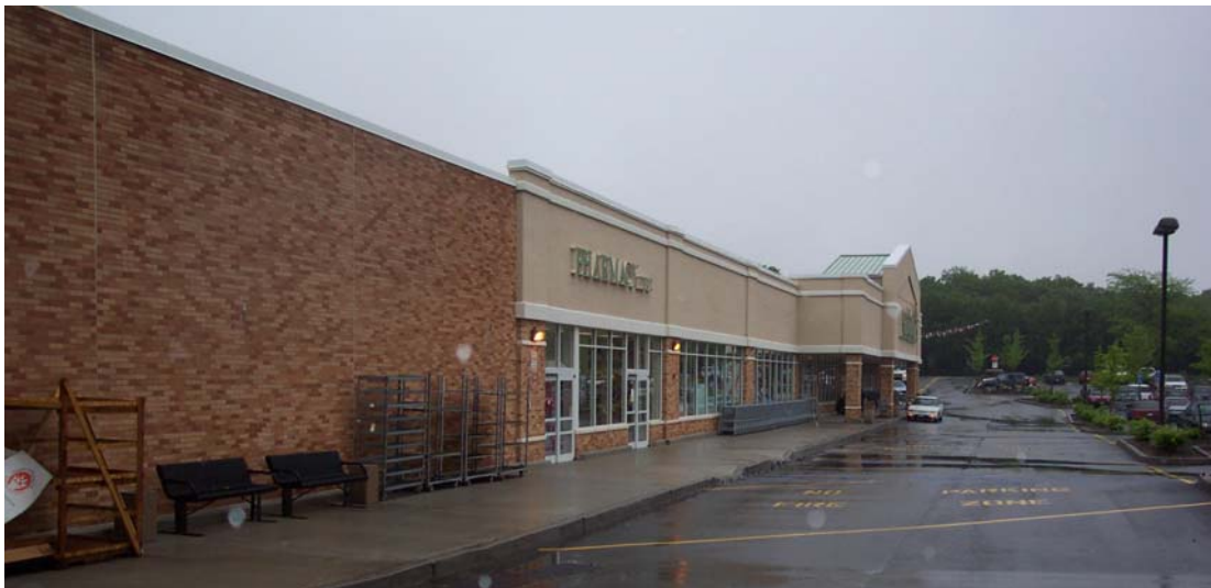
Front of Building (Southwest)
