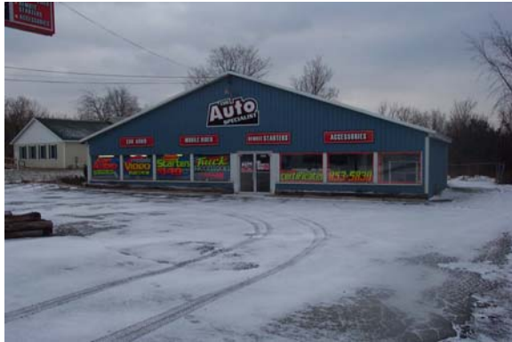
Main Entrance (North)
