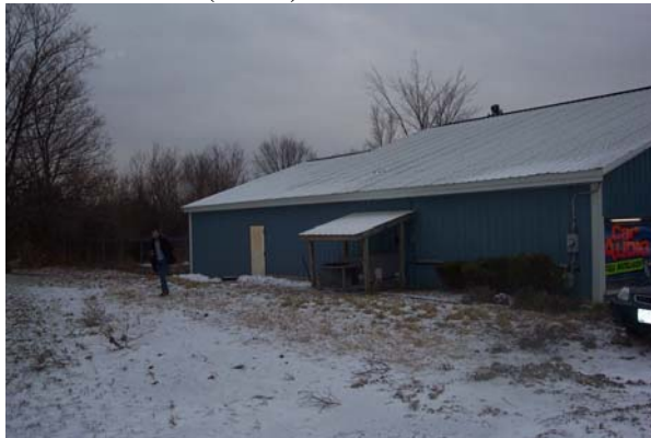
East Side of Building
