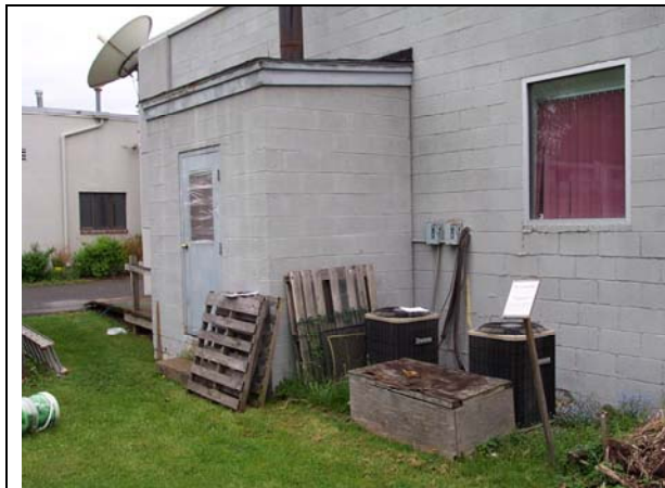
“Furnace Shed” on back of Ag Building
