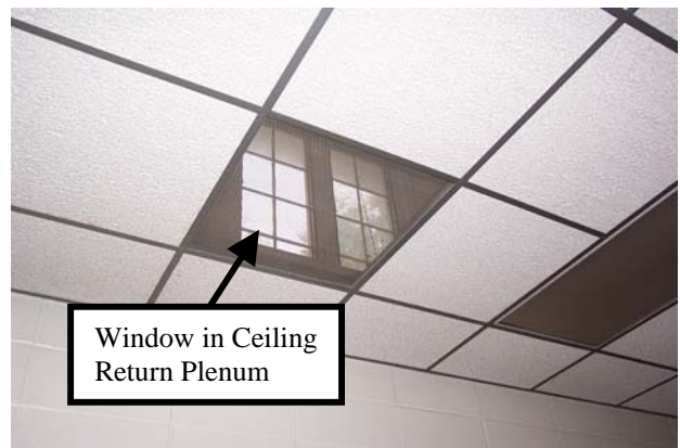
Return Grill to Ceiling Plenum for AC-2
