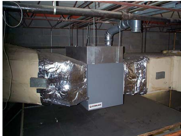
Sterling Duct Heater for Constant Volume Unit
