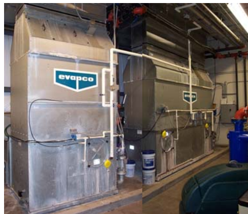
Figure A12-7. Hot Water Boiler and Cooling Towers to Maintain Water Loop Temperature
