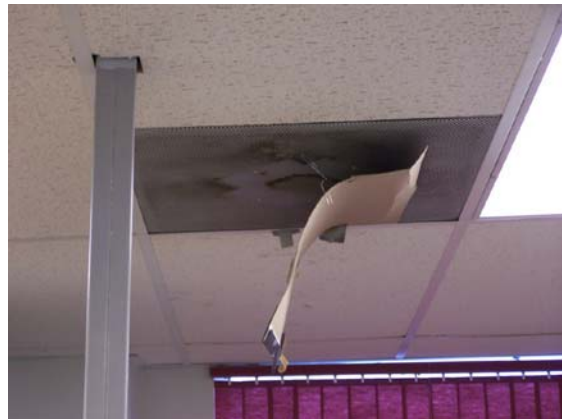
Measured flow – 114 cfm
