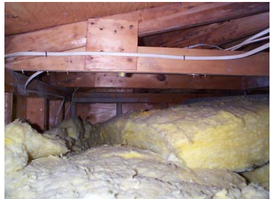
Roof Section at South End of Building
