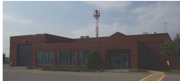
Main Entrance (Southeast)
