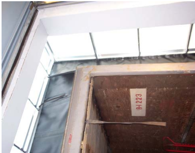
Air-tight Loading Dock with Trailer in Place
