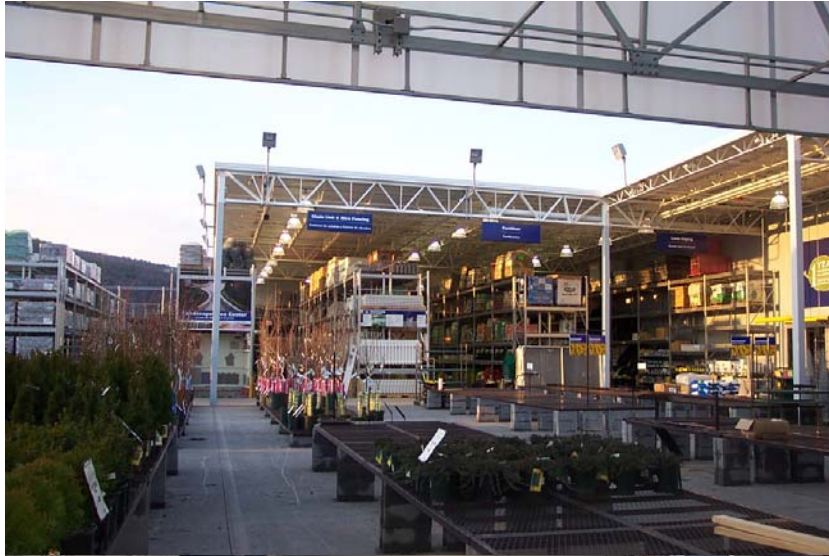
Covered and Uncovered Areas in Outdoor Garden Section.
