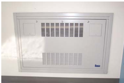
Wall Heater Unit (Used in Vestibules and Bathrooms) Rittling Model: RFRWI-350
