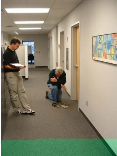
Taking pressure readings under a closed office door (Site 12)
