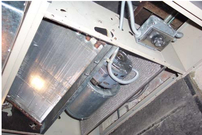
Figure A17-8. Steam Convactor Unit with Fan
