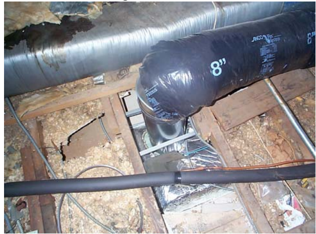
Typical Diffuser Installation
