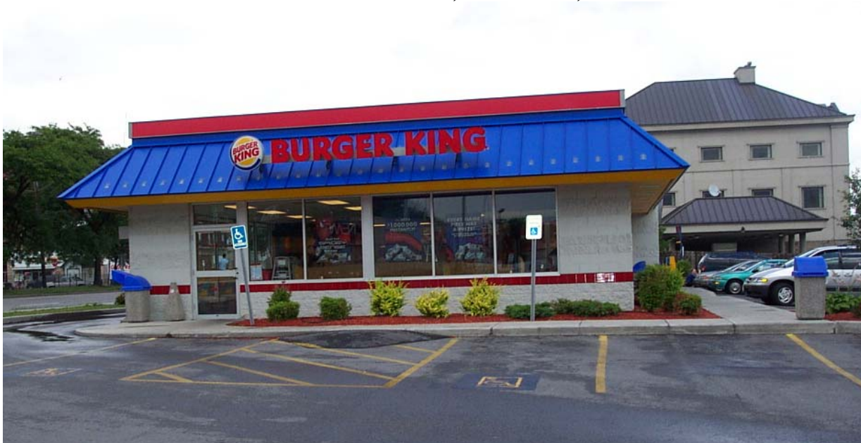
Figure A7-1. Photo of Building (Southwest)
