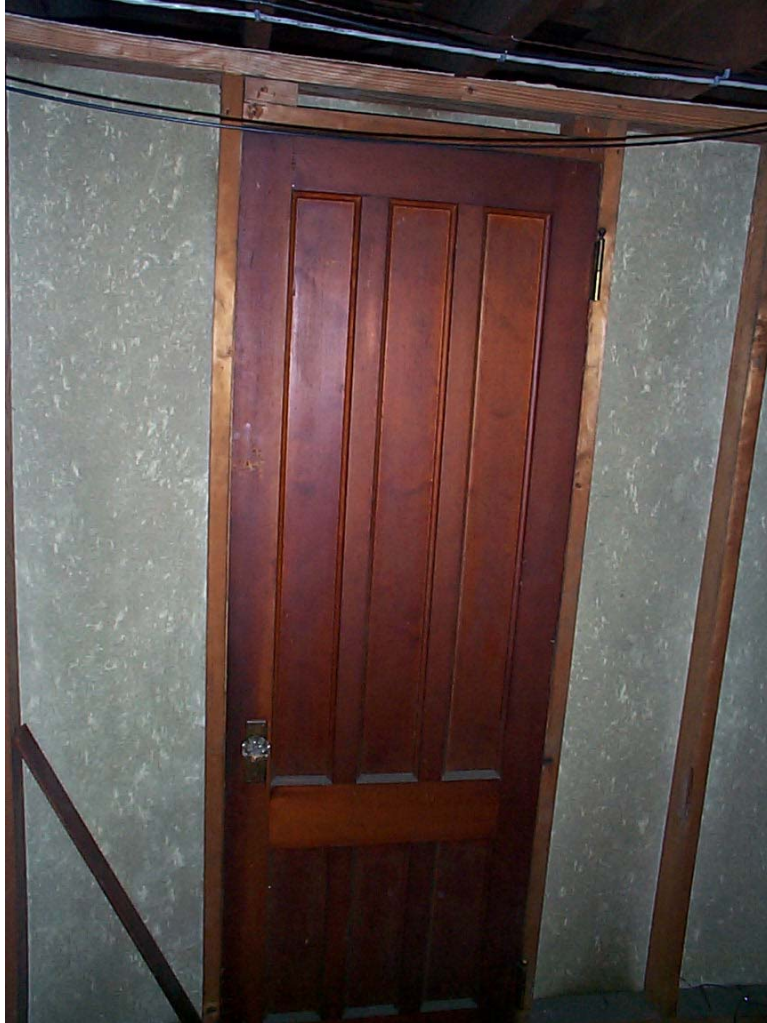
Figure 3-15. Exterior of Elevator Mechanical Room (Viewed from Attic)
