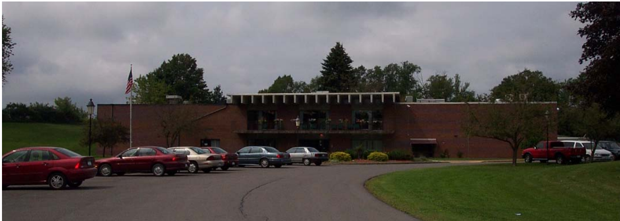
Front of Building
