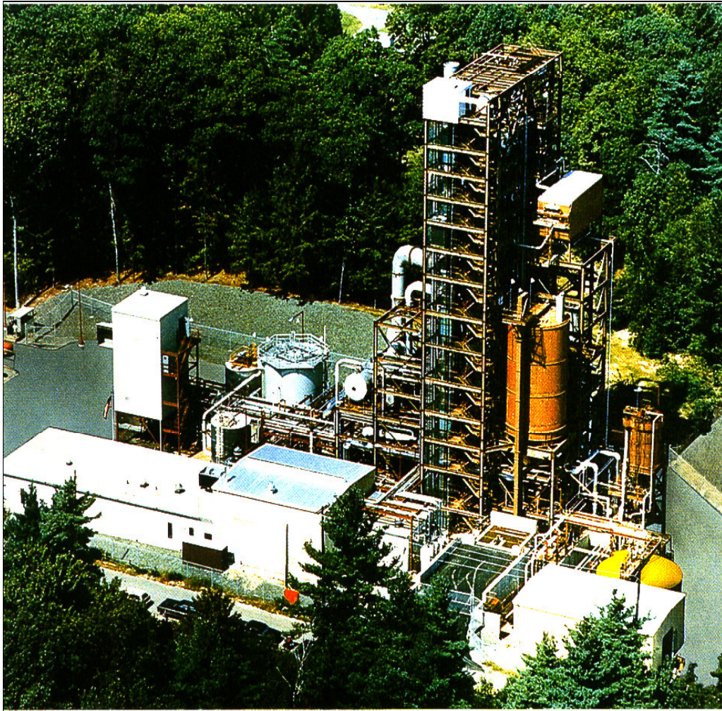
Figure 3-1 - The Windsor Connecticut Coal Gasification Pilot Plant.
