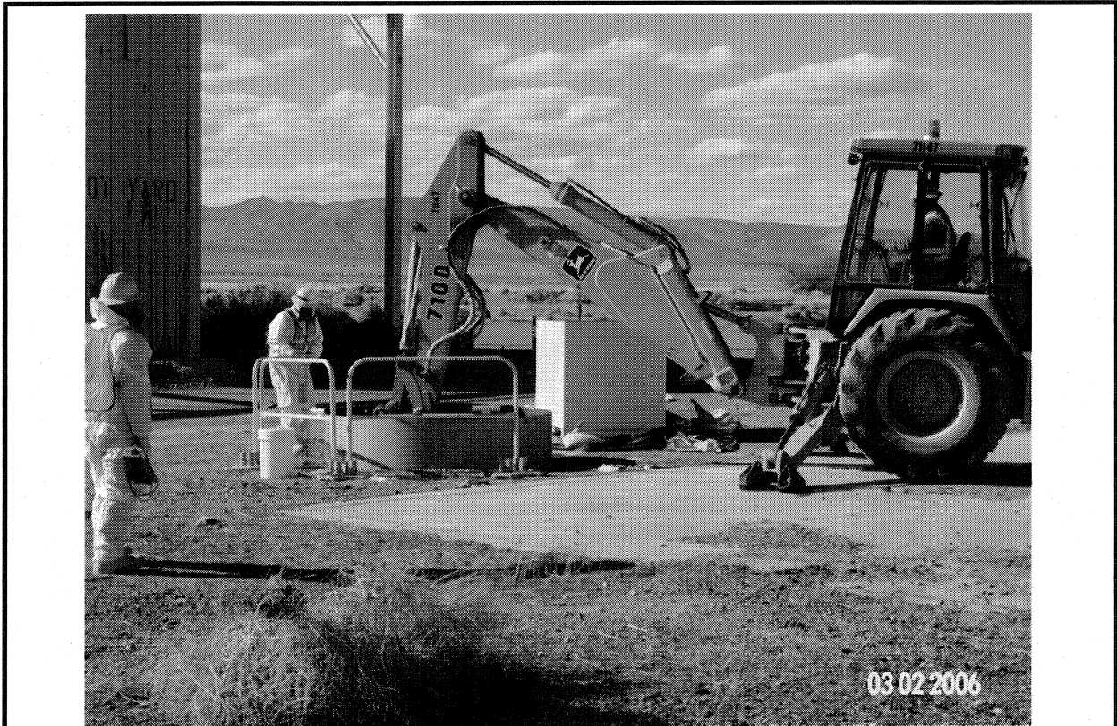
Photograph 5: CAS 03-20-05 Injection well during soil excavation. (03/02/2006)
