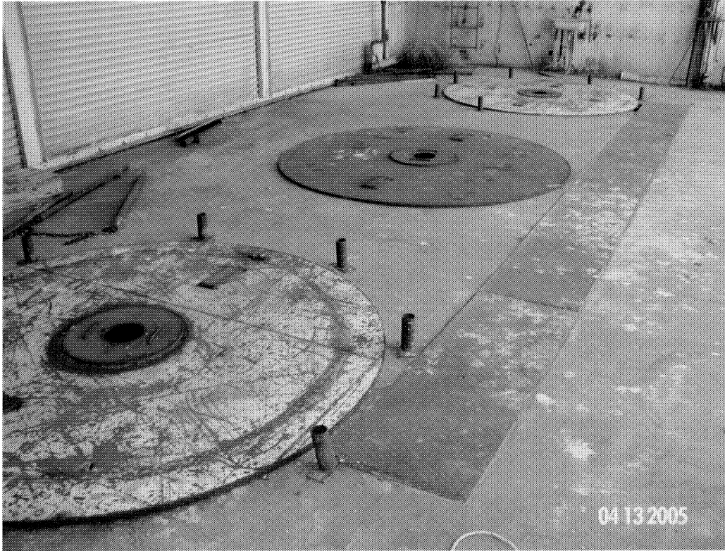
Photograph 1: CAS 03-20-05 Holding tank covers / trenching before closure. (04/13/2005)
