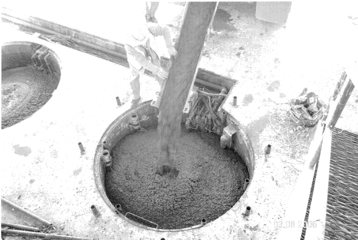
Photograph 2: CAS 03-20-05 Holding tanks / trenching during corrective action. (03/08/2006)
