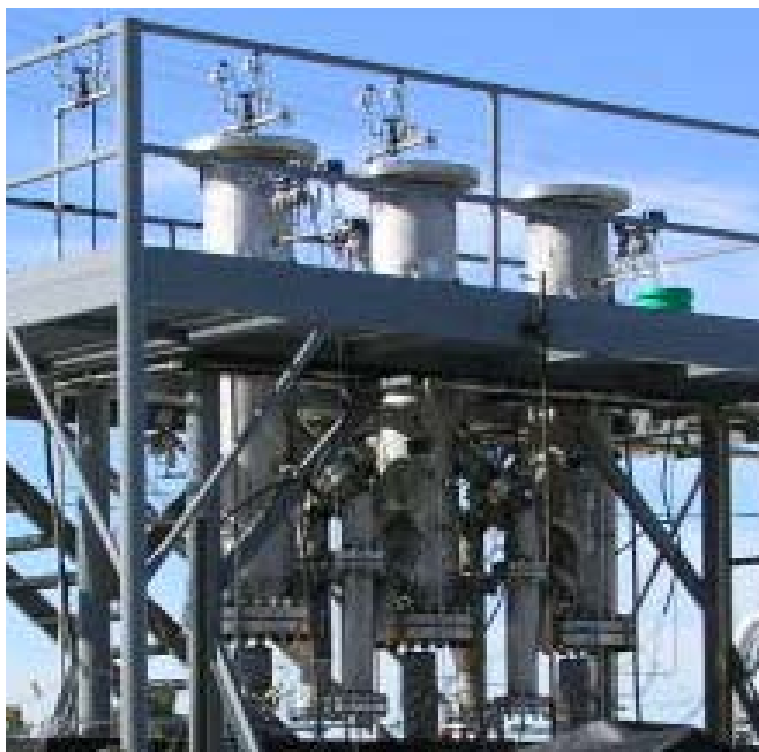
Figure 2-11. Assembled pilot-scale reactors on stand.
