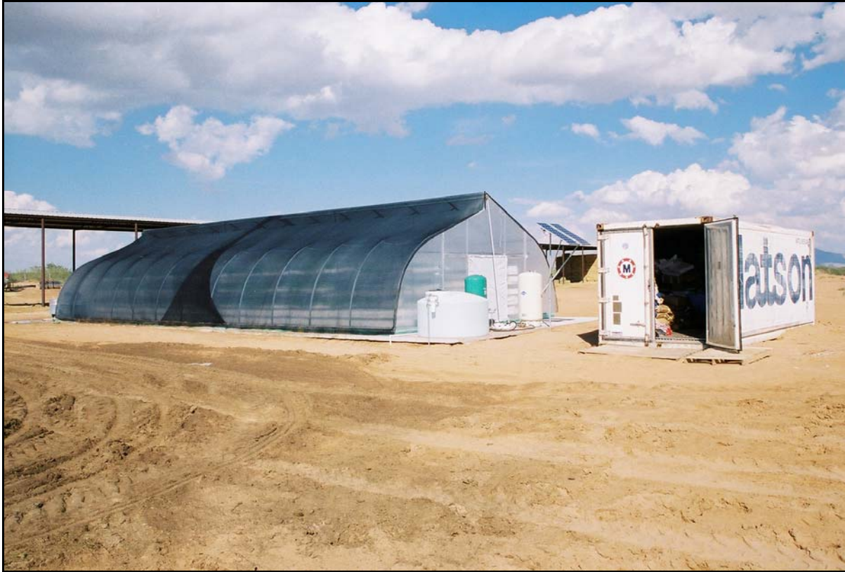
Figure 1-5 Hydroponic forage greenhouse project system built in Santa Teresa, NM. Greenhouse is covered with plastic glazing material and shade-cloth (50% shading) to reduce interior light intensity and overheating. Structure on right is a surplus 20 x 8 x 8-foot double-insulated refrigeration transportainer with stainless steel interior and lock for secure on-site storage of seed, equipment, and other supplies.
