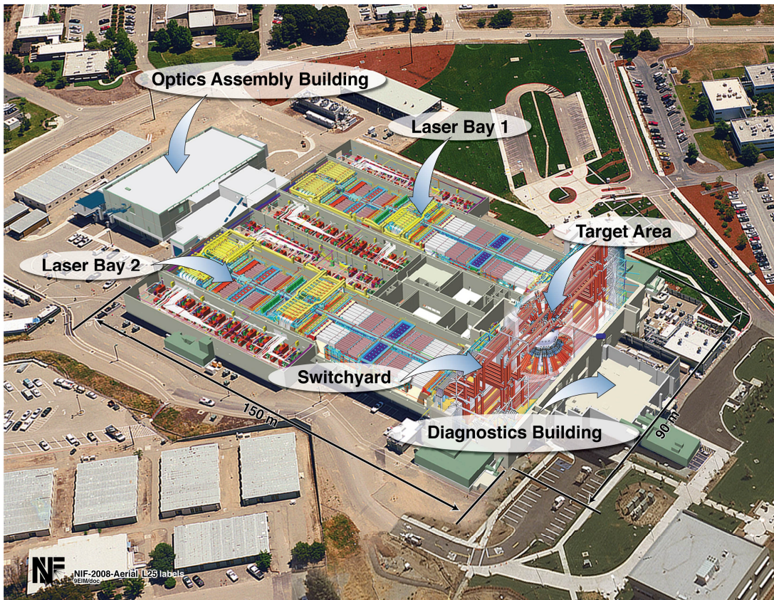
Figure 1: NIF aerial view, showing the two laser bays, switchyard, target chamber area, diagnostics building, and optical assembly building.
