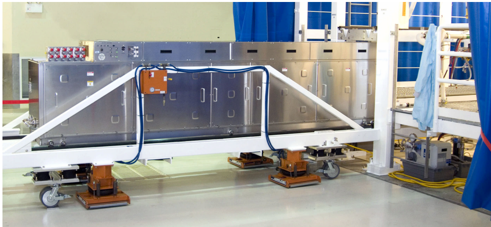
A PAM being installed into NIF laser bay.
