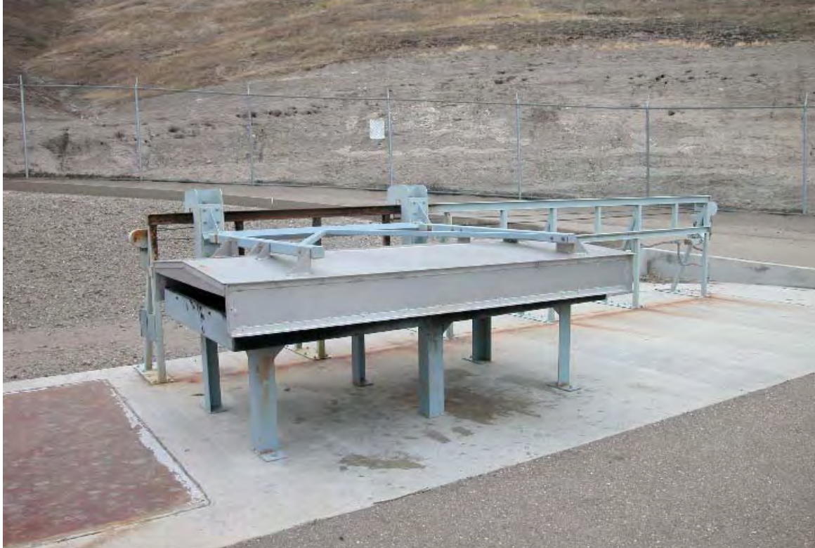
Figure 3. EWTF burn pan, covered. (UCRL-Photo-213179, July 16, 2005)
