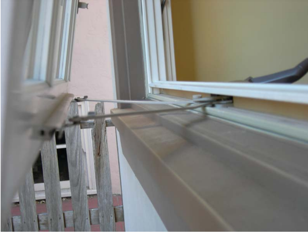
Figure 1. Hardware for window operation is not currently modeled when evaluating window heat transfer. However, hardware often replaces solid materials, is often made of highly conductive metal, and can be a major frame penetration. As window frames become more insulating, such thermal short-circuits can have a significant impact on the overall U-value.
