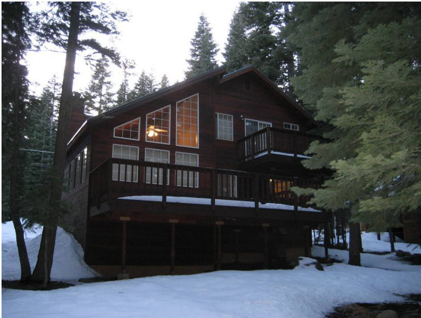
Figure 1. Leaky home in cool climate of Lake Tahoe, CA.
