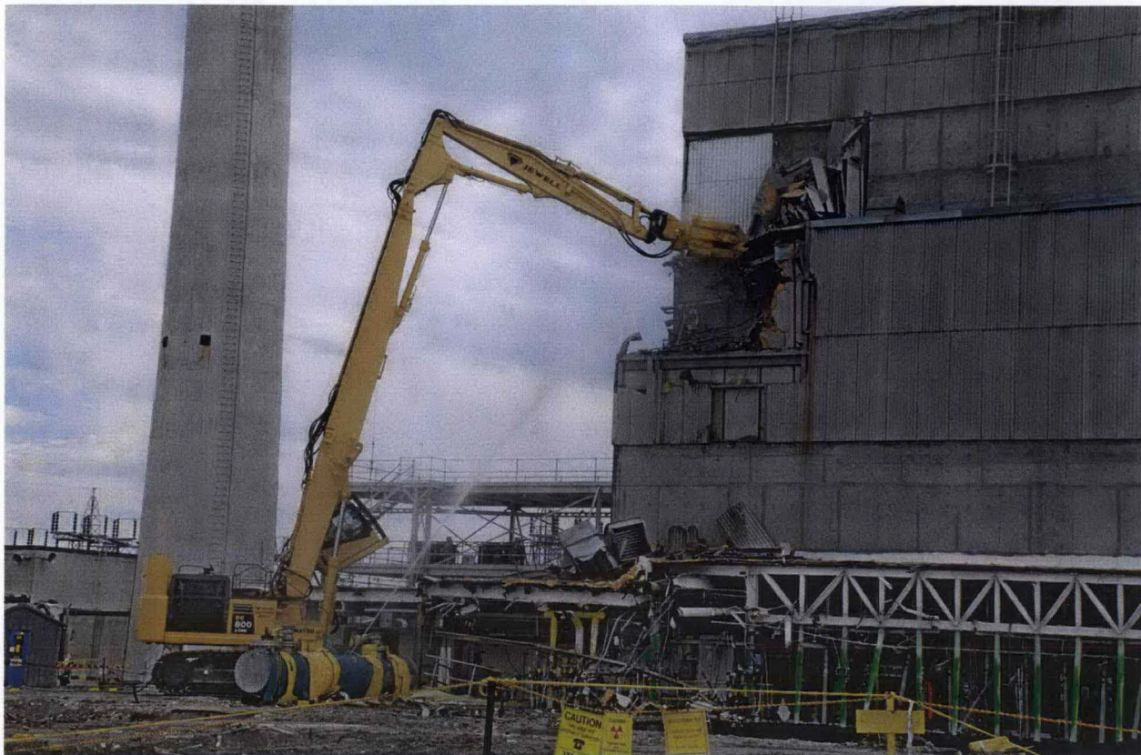
Fig. 3. A high-reach excavator was used to demolish the F-G (reactor interface area) area.
