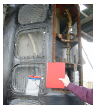
Exterior Forward Sail Cover Plates Removed
