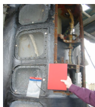
Exterior Forward Sail Cover Plates Removed
