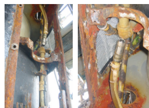
Internal Forward Sail Corrosion
