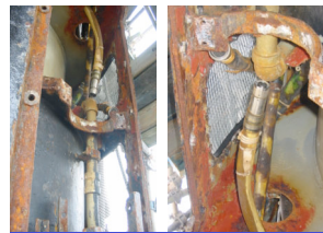
Internal Forward Sail Corrosion
