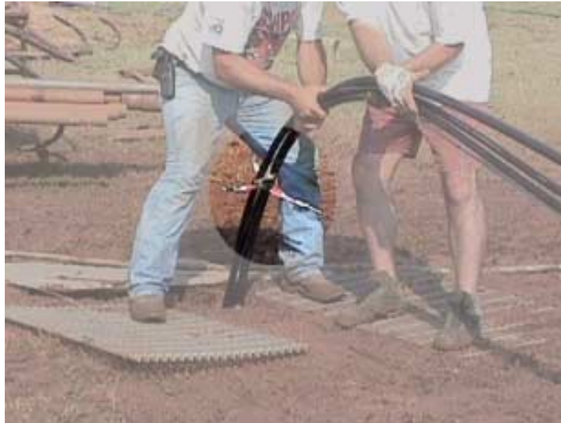
Figure 1a. Thermistor system during installation.
