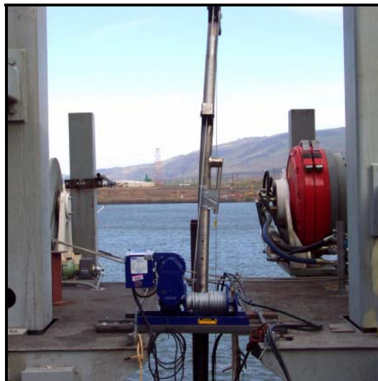
Figure 3.9. Electric Hoist and Davit System Used to Deploy the DIDSON
