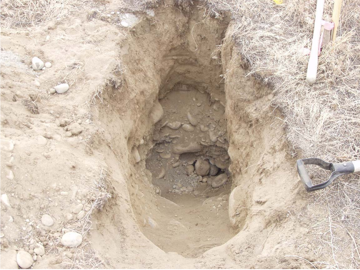
Figure 9. Soil Sampling Pit Used for Collecting Near Surface (<1-m) Grab Samples. Note the abundance of gravels and cobbles beginning at a depth of approximately 0.75 meter.
