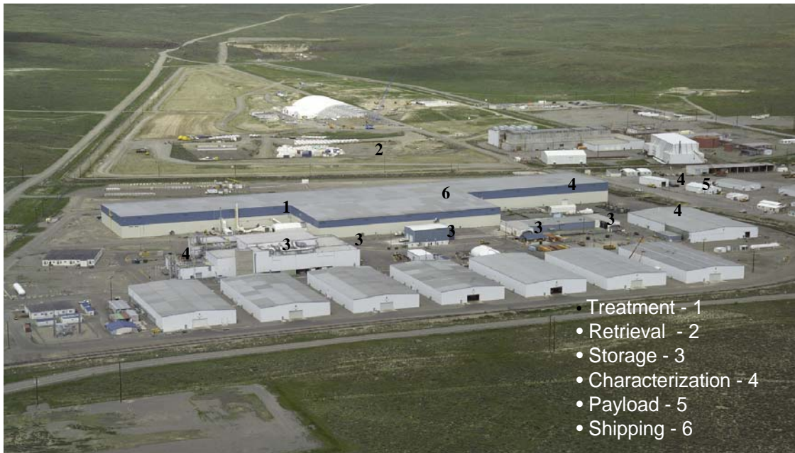
Photo 1. Advanced Mixed Waste Treatment Facility
