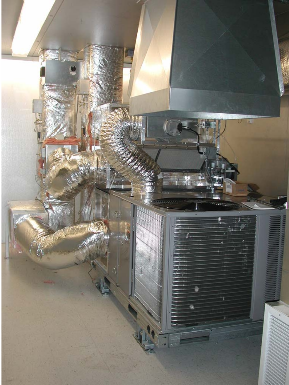
Figure 7.20. View of the completed integrated EERV/rooftop unit.
