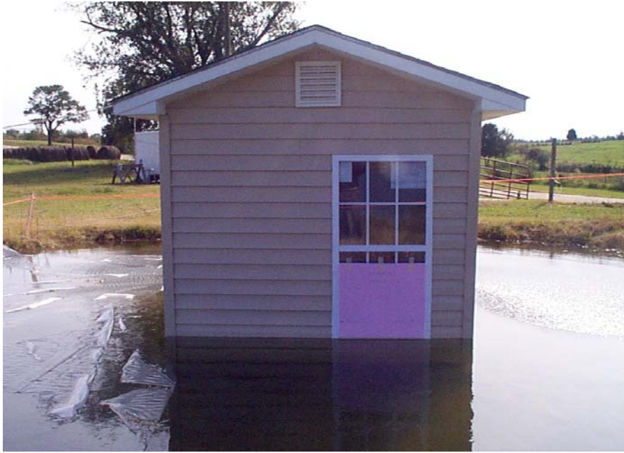
Figure 6-2 Module S-3 Wall 1. Dam on window during flooding is staying in place.
