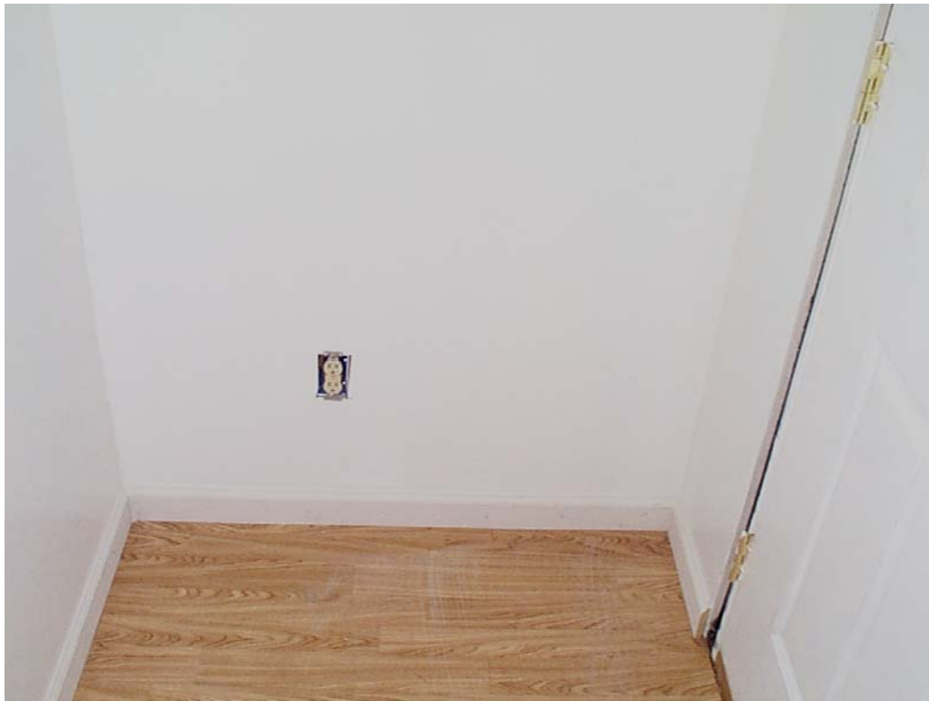
Figure 6-11 Module C-3 (Wall 2) Pre-flood. Walls and floor in new condition
