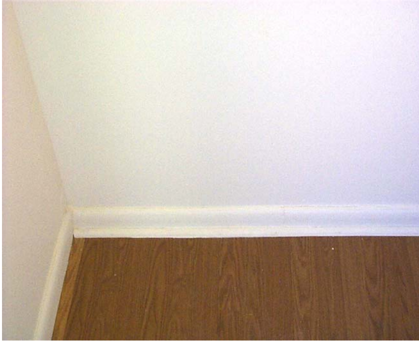
Figure 5-4 Module S-2 (Wall 4) Pre-flood. Walls and floor are in new condition.
