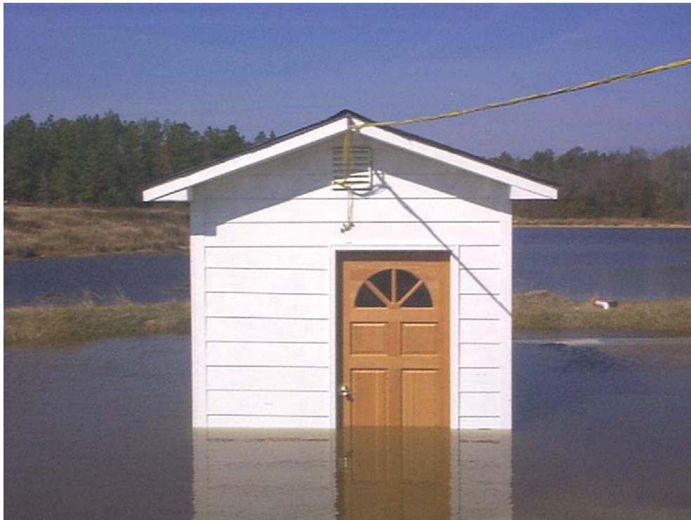
Figure 3-7 8 ft x 8 ft slab on grade module during flooding
