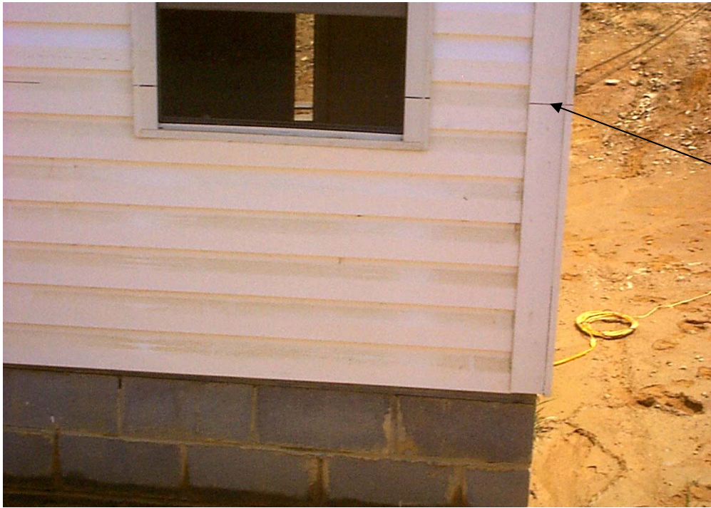
Figure 5-16 Module C-2 (Wall 1) Day 8 before washing. Wall is discolored
