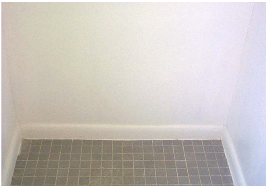
Figure 5-9 Module C-2 (Wall 2) Pre-flood. Wall and floor in new condition
