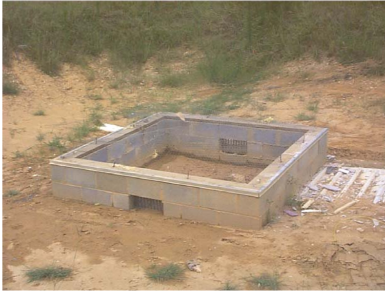
Figure 3-3 Crawlspace concrete block stem wall foundation located in test basin
