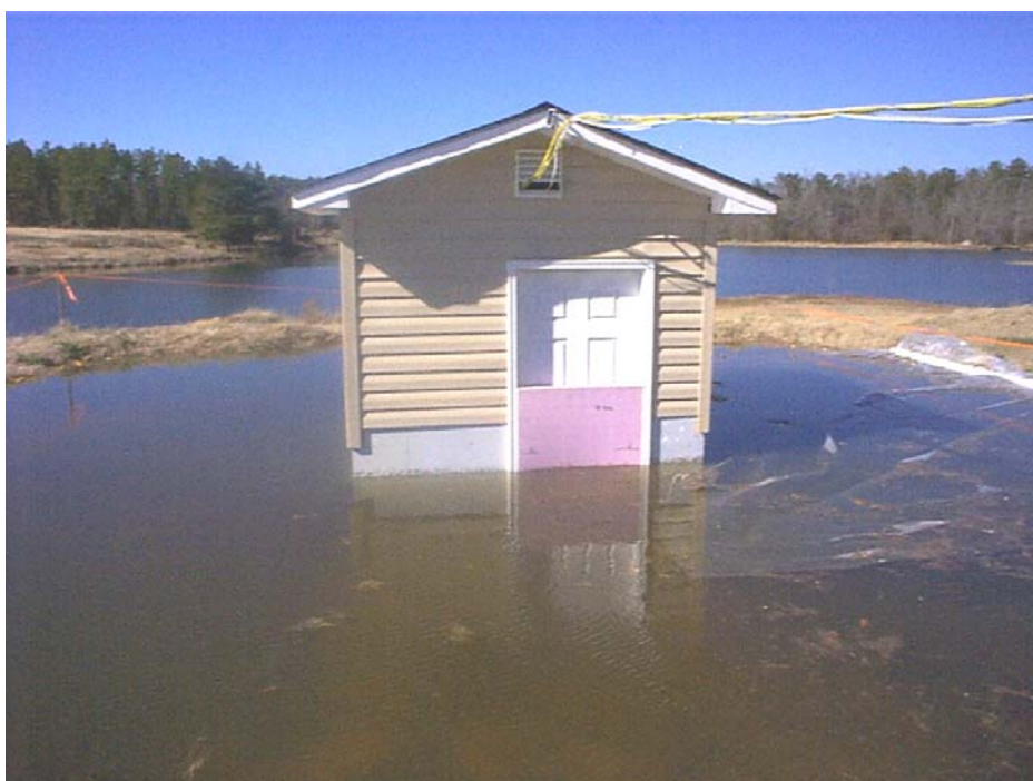
Figure 6-34 Module S-3a South wall during flooding. Note the inward deflection of the flood dam at the door. This indicates a significant differential in water level (outside to inside) at the time of the photograph.
