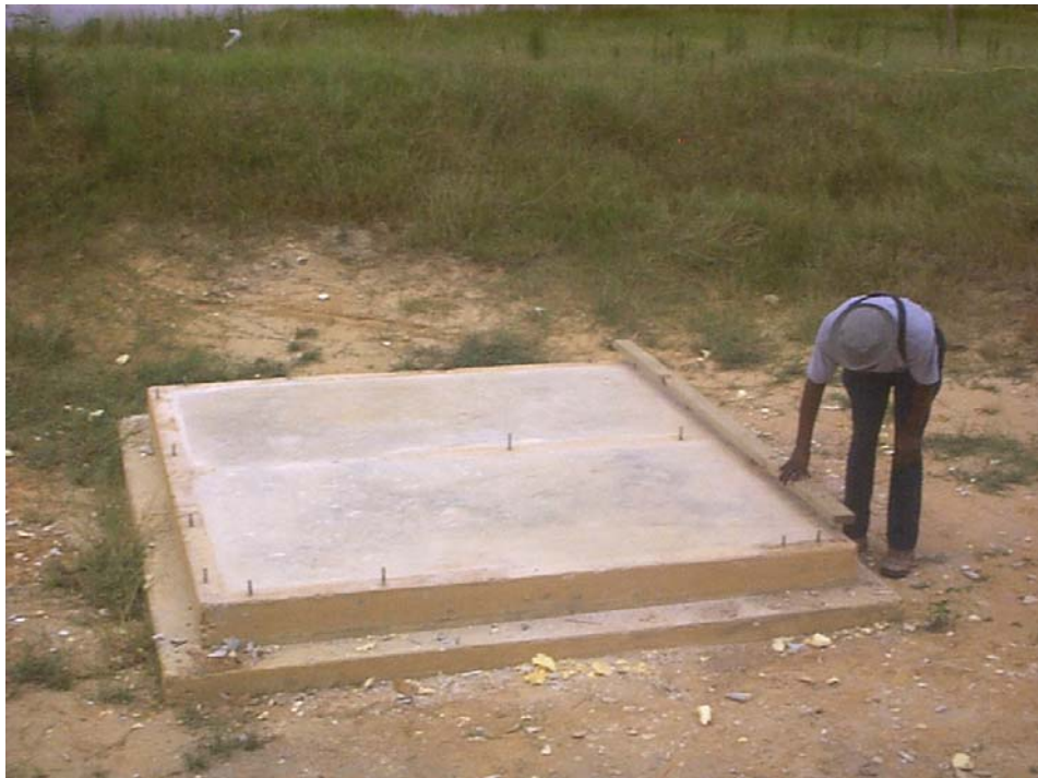
Figure 5-19 Module S-2 - Foundation of module at demolition
