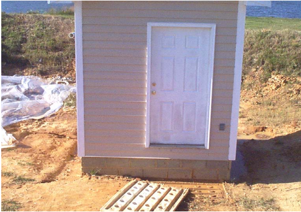
Figure 3-6 8 ft x 8 ft crawl space module before flooding
