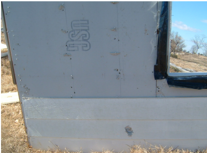
Figure 6-38 Module C-3, Wall 1, Exterior. No mold or severe staining was observed at autopsy which occurred 15 months after the flood test. The flood level was about 6” above the windowsill in this photograph.
