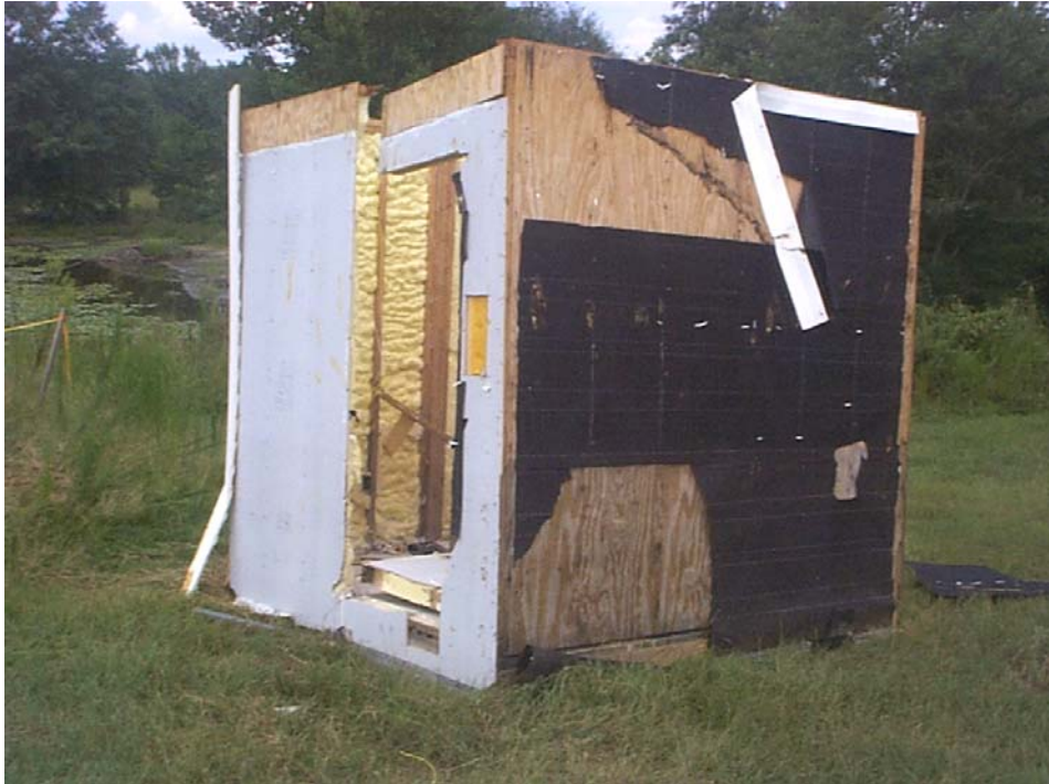
Figure 5-18 Module C-2 - Body of module at final autopsy and demolition
