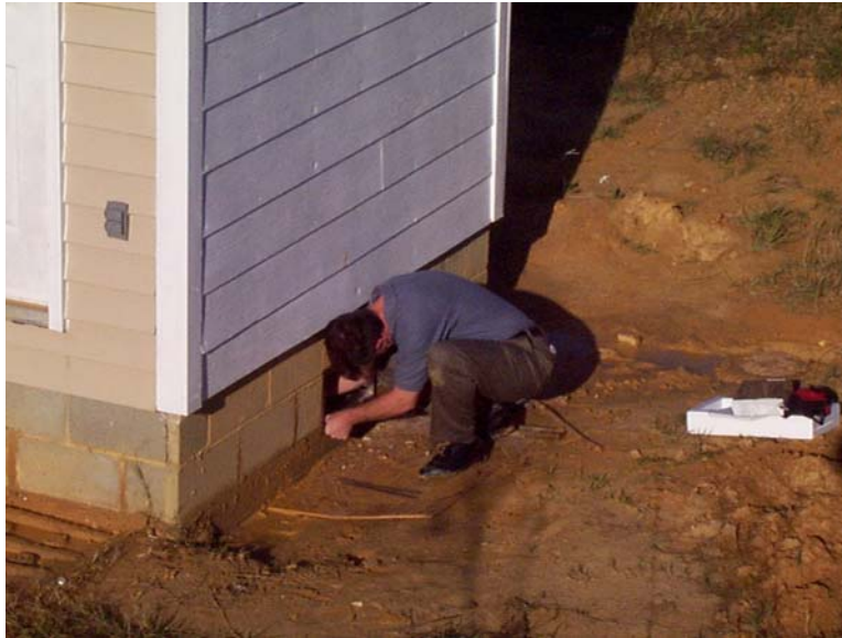
Figure 6-4 Installing an operable flood vent in Module C-3
