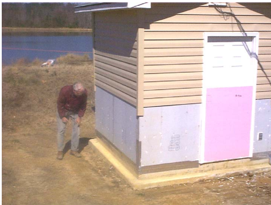
Figure 6-33 Module S-3a, south and west walls being inspected. Before flooding
