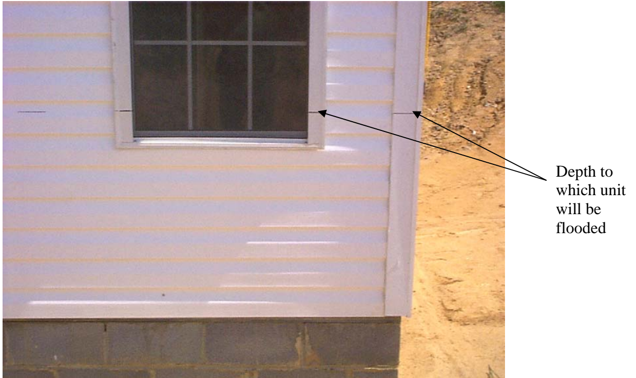
Figure 5-14 Module C-2 (Wall 1) North wall, Pre-flood. Wall is in new condition
