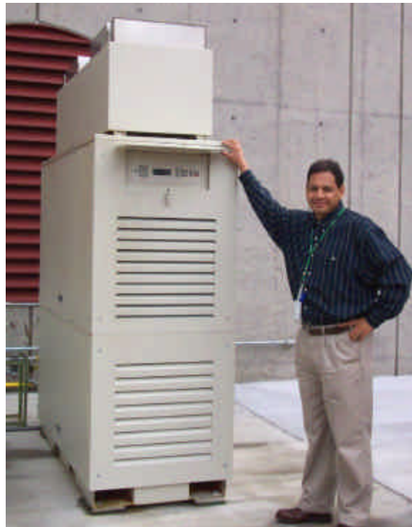
Capstone microturbine - 60 KW
