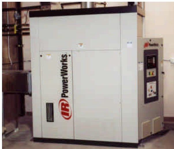
Ingersoll Rand's microturbine makes use of a high-speed gearbox instead of a high-frequency power converter
