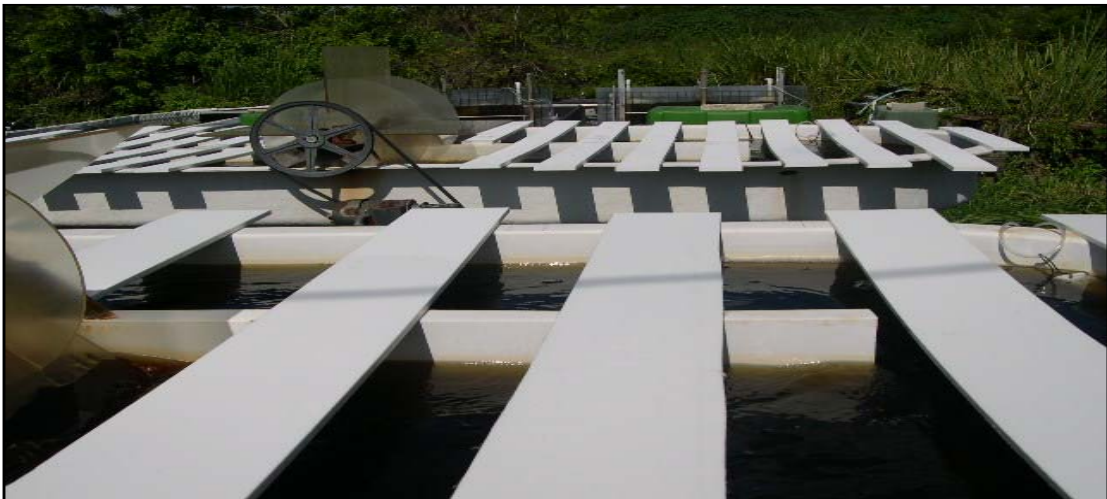
Intermittently Illuminated Raceway Pond, 55% Open Area (15cm wide slat, 15cm wide gap)
