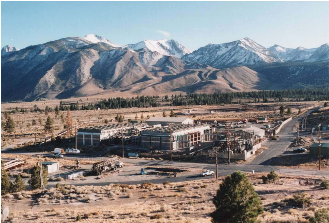
Figure 3. Mammoth Pacific L.P.'s geothermal power production plant near Mammoth Lakes, California where silica extraction R&D is currently being carried out.
