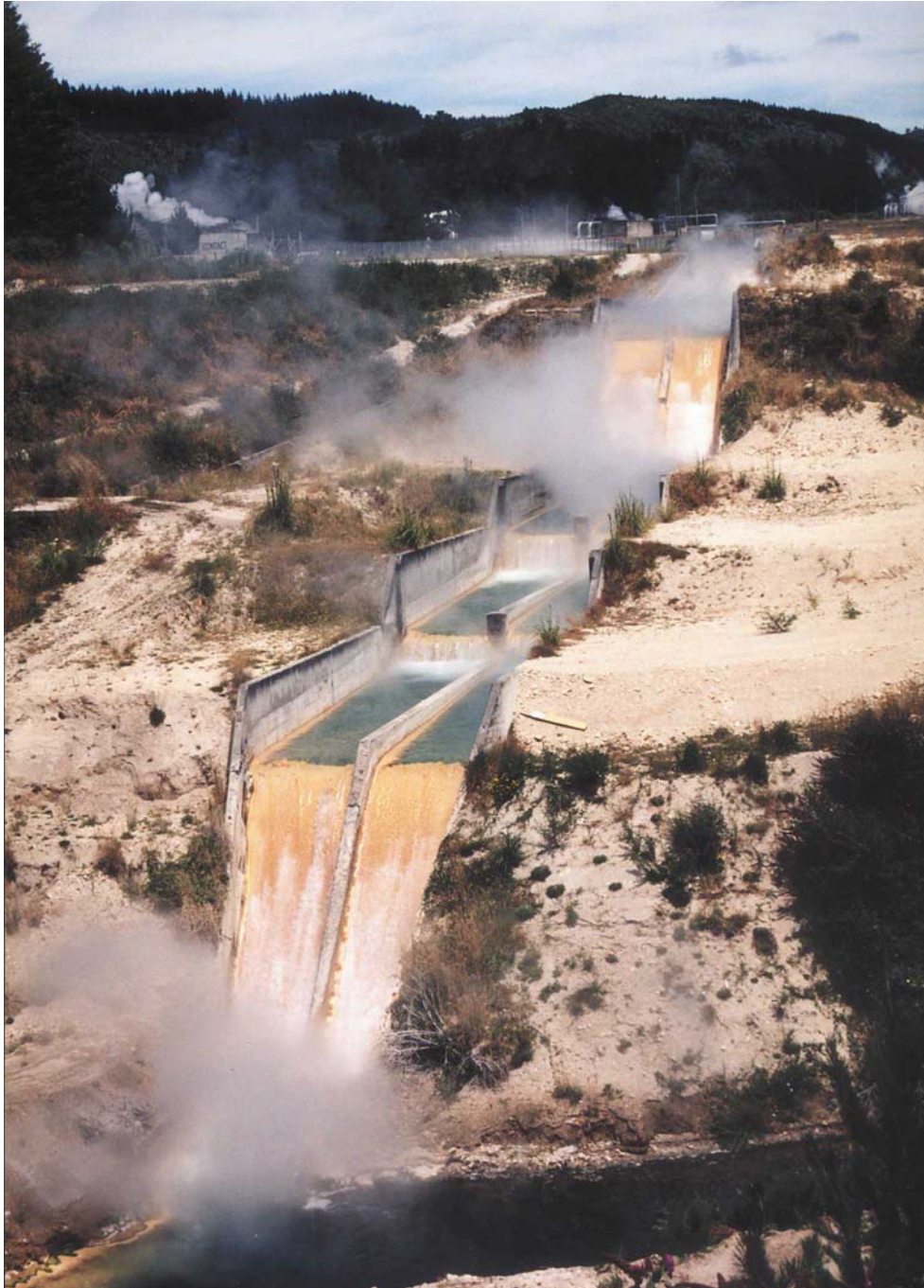
Figure 1. Geothermal fluid drain at Wairakei, New Zealand geothermal site. Silica precipitates of orange-brown color line the channels. A bluish color indicates the presence of colloidal silica in the water.
