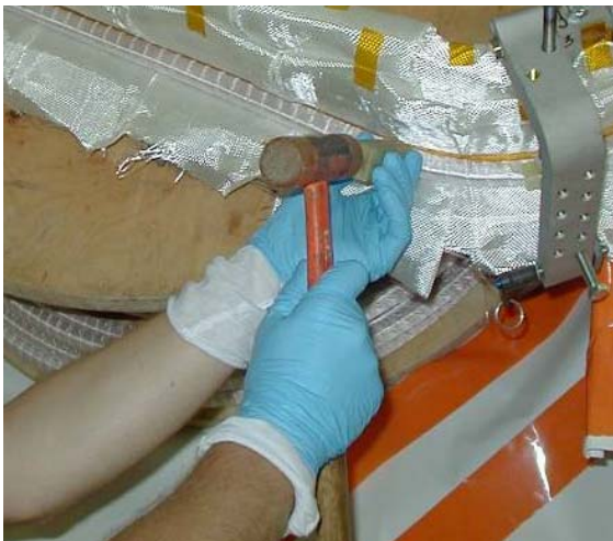
Figure 3- Setting Turns in Position
