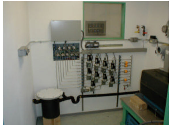
Fig. 2. Module with gas distribution system.
