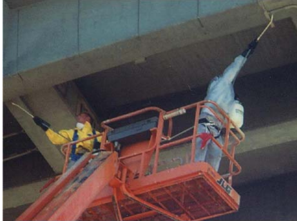
Figure 5 - Spraying humectant on the Yaquina Bay Bridge.
