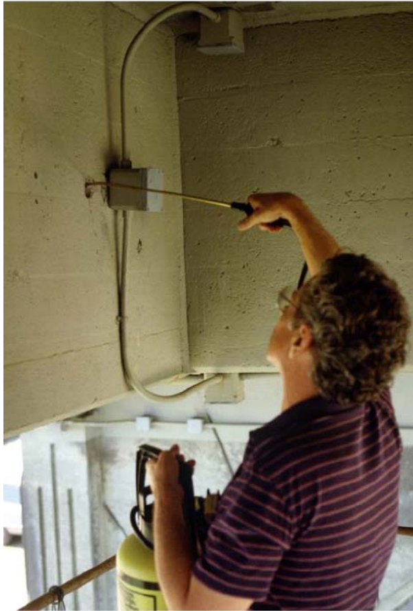
Figure 7 - Carbon anode coating on the north end of the Yaquina Bay.
