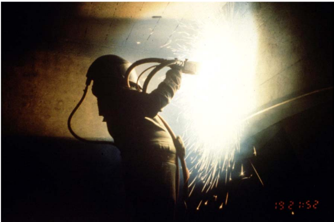
Figure 2 - Thermal spraying using the twin-wire arc spray process.
