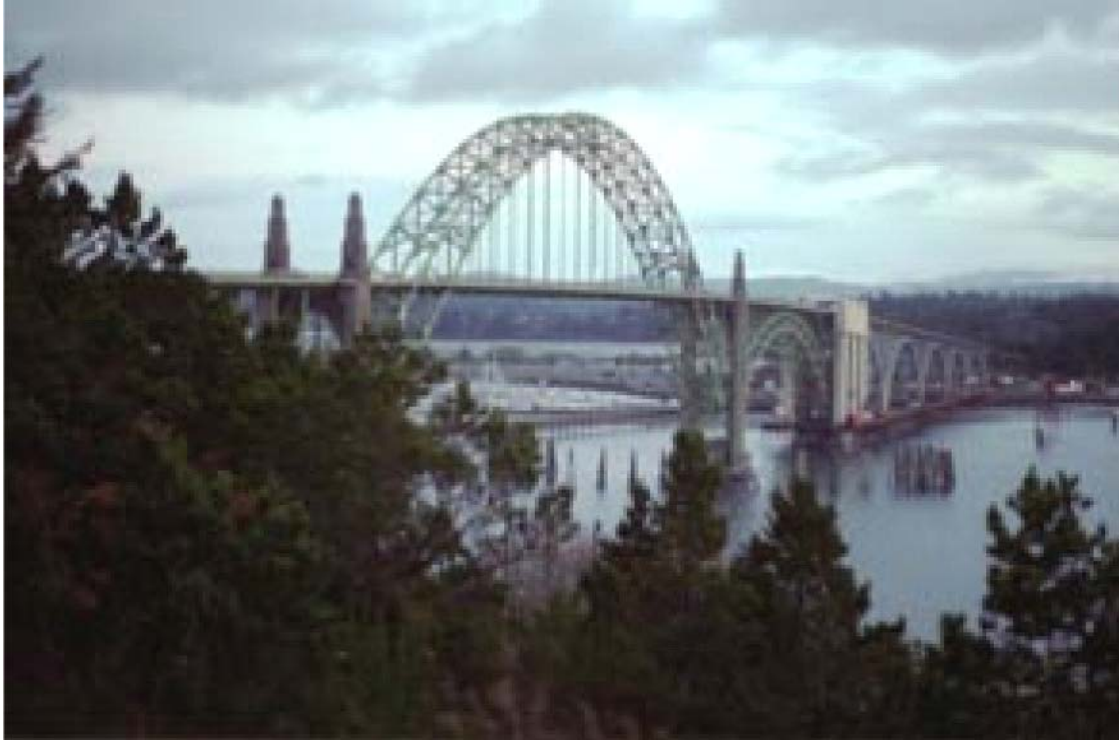
Figure 1 - Yaquina Bay Bridge built in 1936 and located on the Oregon Coast at Newport.
