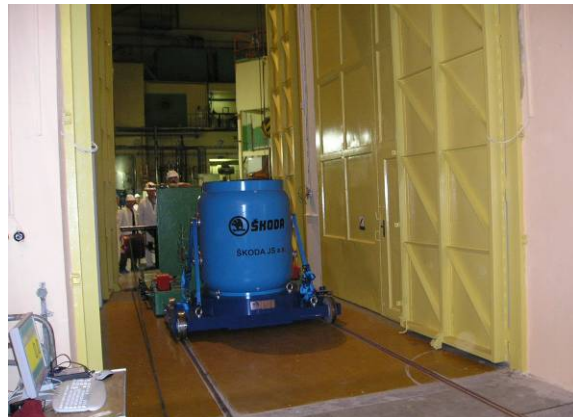
Figure 5. The VPVR/M cask being moved into the Away from Reactor storage area.
