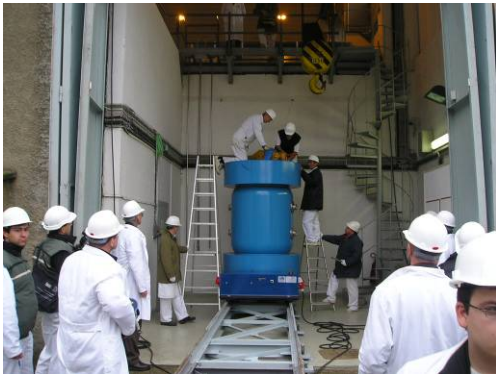
Figure 7. Cask transfer device on rails into the High-Level Waste Storage Facility entrance hall.
