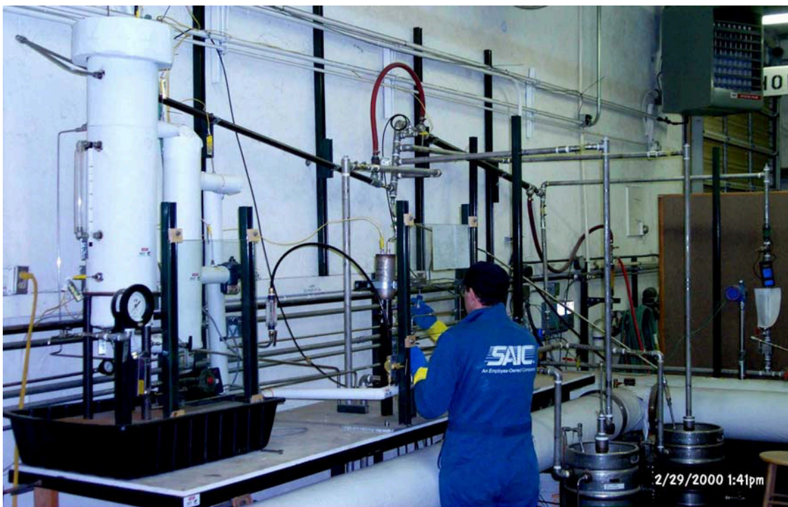
Figure 3-1: STAR Center Bench-Scale Evaporator System
