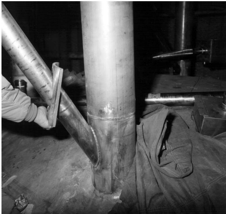
Figure A-6. Typical vessel connections on bin in the Calcined Solids Storage Facility V (81-851).
