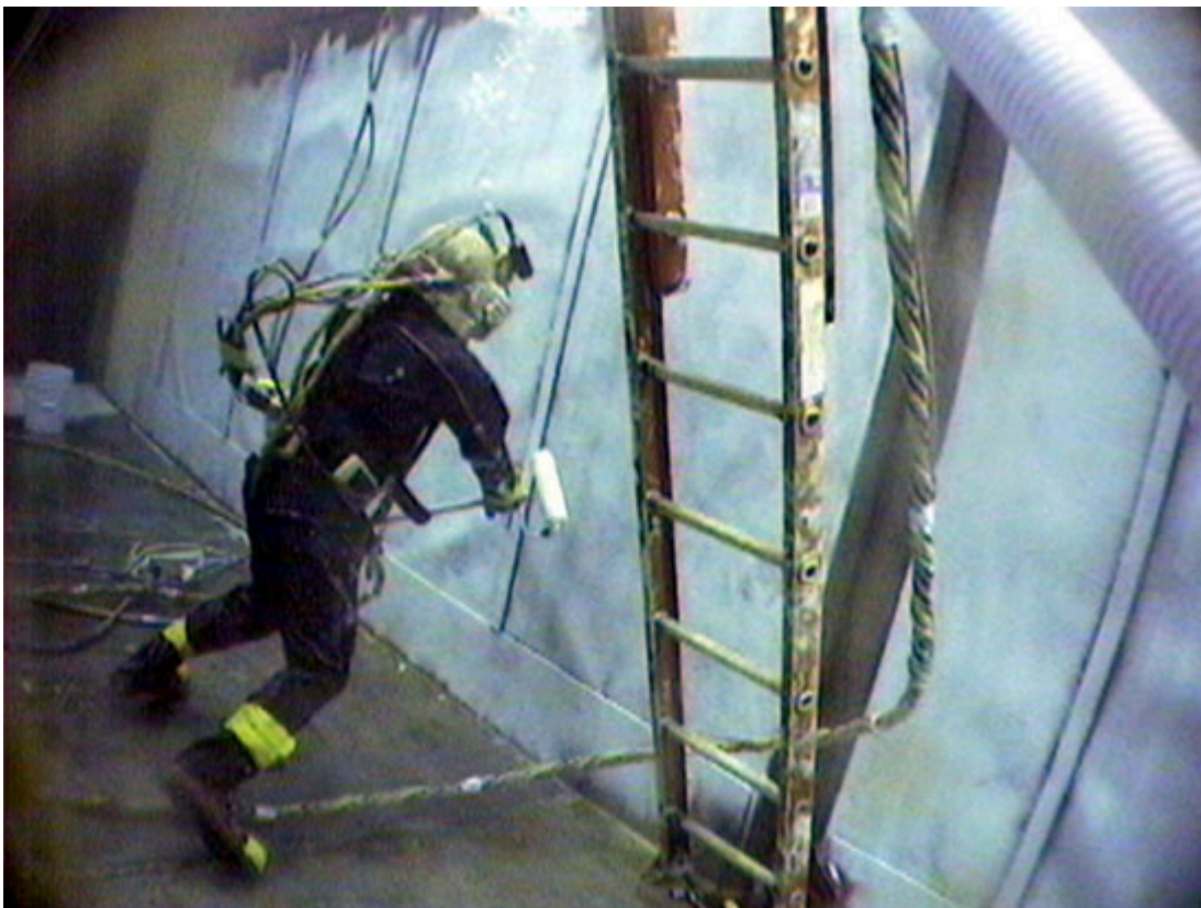
Applying fixative to the wall of the MTR canal.
