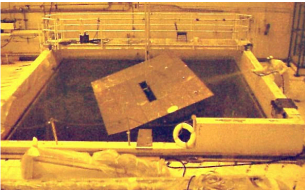
Debris and equipment removed from basin
