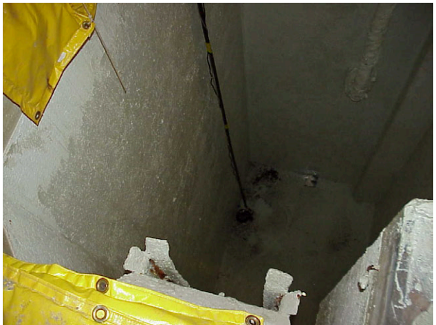
CPP-603 Overflow Pit
