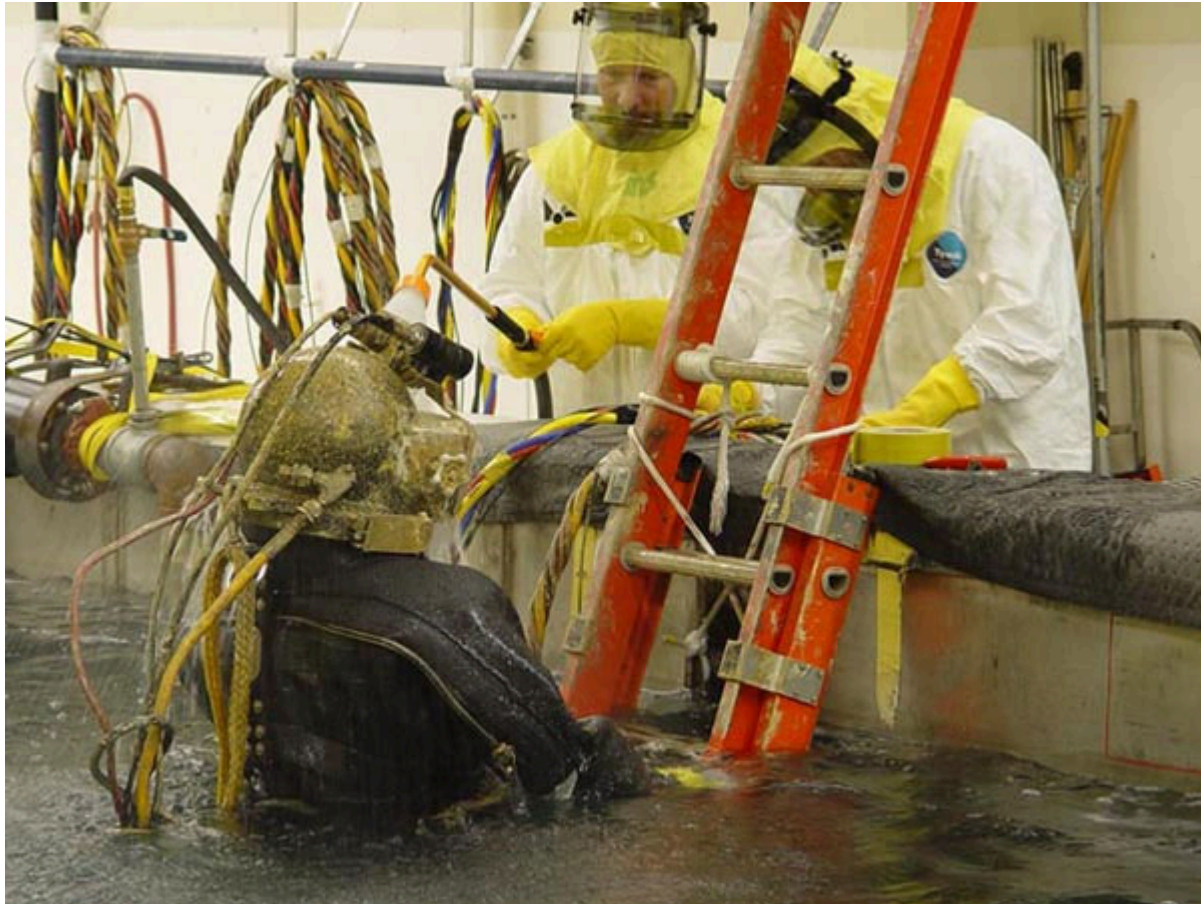
Dive tenders spray a diver as he emerges from the water for contamination control.
