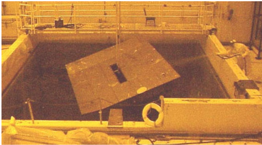
The transfer cart is removed from the basin vestibule in the TAN hot shop.
