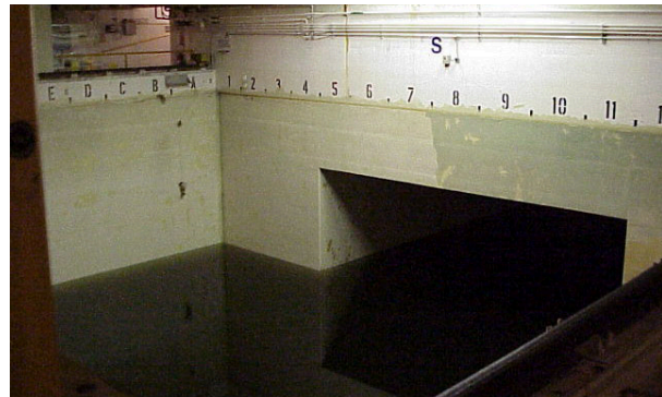
Water removal under way (Water darkened by calcium hypochlorite)
