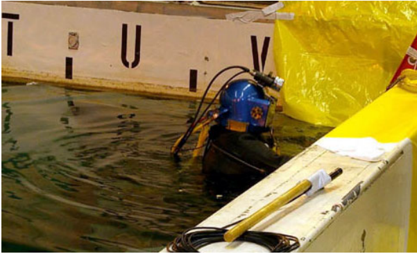
Divers enter the basin to begin cleaning
