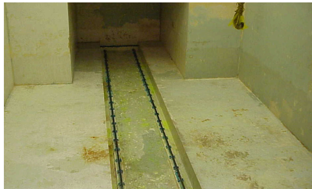
Water removal complete
