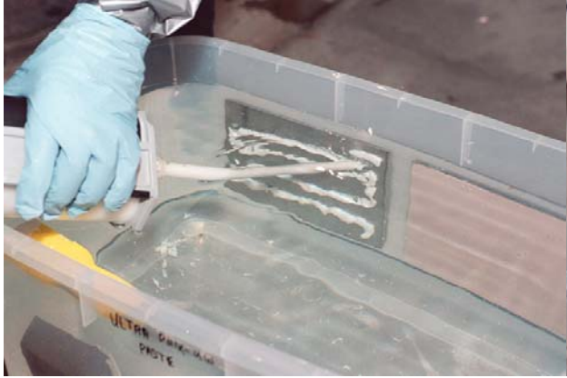
Applying Ultra Phix-UW to the stainless steel with special mixing gun.
