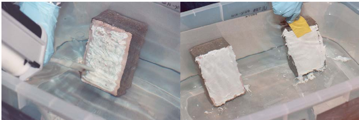
Applying Ultra Phix-UW to the epoxy coated brick with special mixing gun.
