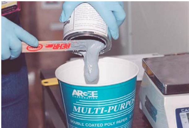
Corro-Coat FC 2100 was relatively easy to mix.
