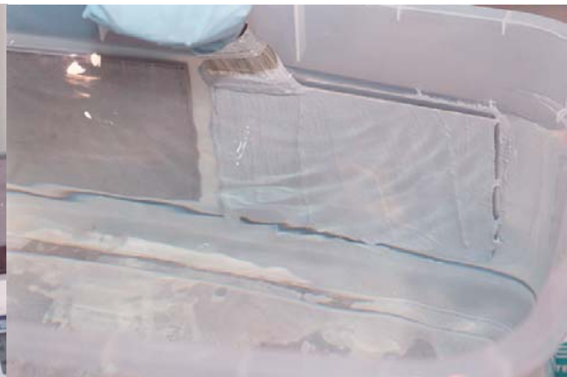
Corro-Coat FC 2100 was applied with a brush.
