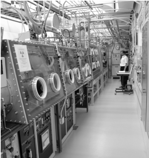
Fig. 1. AFCI glovebox in the Fuel Manufacturing Facility at INL.
